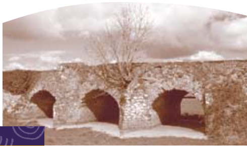
Bridge of the Maudelynes The oldest bridge in Duleek
