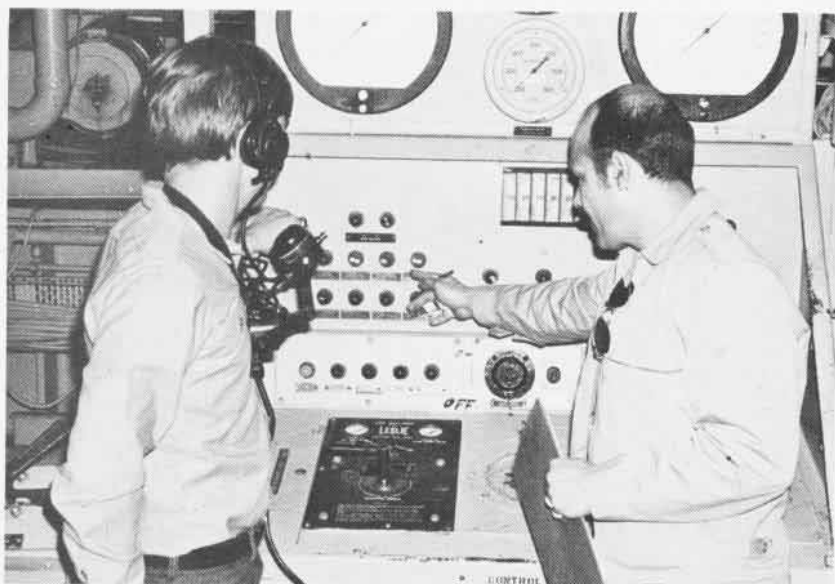
ABF1 Padgett shows AA Collum how to use the AEL-MK3 solid contamination fuel tester, top left. Students become acquainted with the A-4 launch sequence, top. Below decks in the TAP, AA Sherwood receives instruction in using the catapult control console from instructor ABEC Ronald L. Fagg, above. AA Carl C. Zaska learns taxiing and spotting evolutions on the TAP, left.
