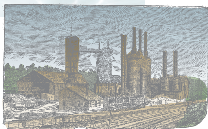
In the summer of 1890, Youngstown extended the city limits to include the Brier Hill Furnaces which were erected by Governor Tod. They had what was called a wash-metal plant where pig-iron was resmelted (Mahoning County, Ohio, Henry Howe).
