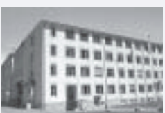
Sainte-Croix, CH heating technology
