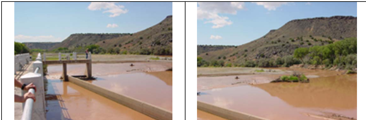
Looking downstream from above diversion eastside of river
