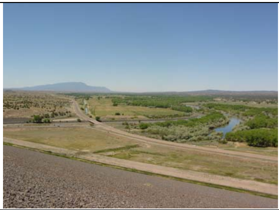
Looking south from dam crest
