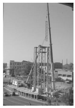
In late October the major steel framing is in place with the steel for the roof yet to be erected. The bell console will be located at the top of the larger framing for the tower base with the bells to be housed in the upper portion of the steel framing. A spiral stair will be placed in the southwest leg of the tower. Visible is a stair in the console room accessing the bell chamber with a ladder yet to be installed in the upper southeast leg to provide access to the attic space.
