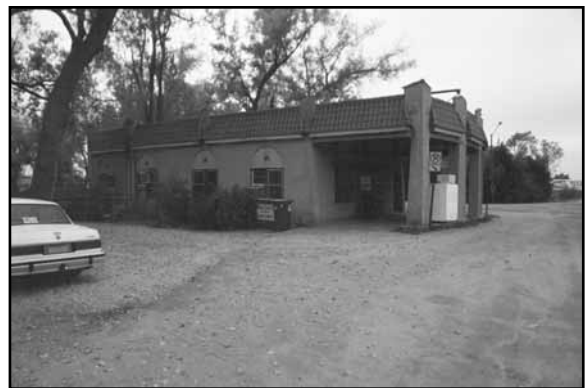
Shady Bend at east side of Shady Bend Road near Grand Island, HL00-033. Former cabin court and tourist complex. Previously determined eligible.
