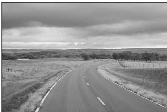
Current view of former alignment of U.S. Highway 20 through Smiley Canyon in Dawes County near Fort Robinson, SX00-34
