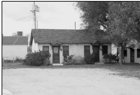
Motel Court at U.S. Highway 20 and B in Valentine, CE14-062
