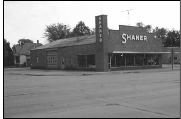
Shaner Motors at the southeast corner of 13th and H Streets in Geneva, FM05-129. One-story, brick auto dealership.
