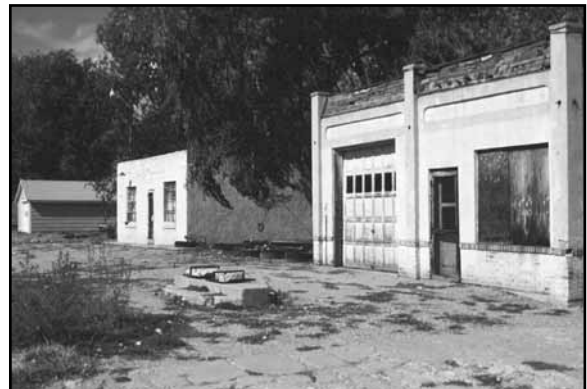
Garage at the northwest corner of Tecumseh and Vinita Streets in Wauneta, CH06-028.
