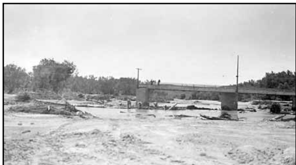
Flooding washes out north portion of Bartley State Aid Bridge on Highway 6 (D-L-D) in Red Willow County near Bartley, 1935 (Photo courtesy of NDOR)
