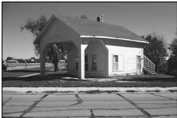
Gas station at 801 East 8th Street in Cozad, DS02-055. Frame, front gable gas station with canopy.
