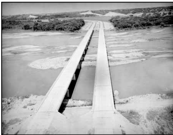
View of Interstate 80 spanning the Platte River from Cass County looking into Sarpy County near Ashland in 1961 (Photo courtesy of NDOR)
