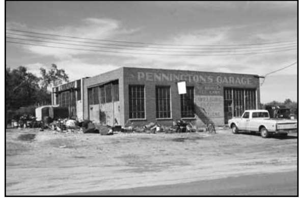
Pennington's Garage at southwest corner of Highway 6 and Tecumseh Street in Wauneta, CH06-021. Brick garage building with industrial metal sash windows.
