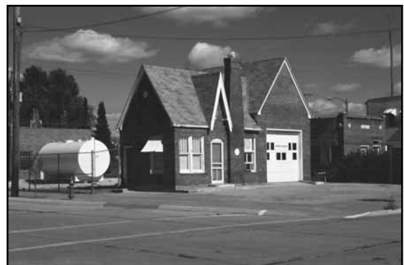
Gas station at northwest corner of Spruce and Highway 30 in Sutherland, LN08-046. Brick, house style gas station. Previously identified and recommended as eligible.
