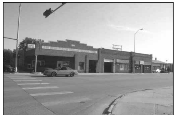
Service station at 1030 West 2nd Street in Hastings, AD04-107. Brick service station completed in 1925 by W.J. Bauer.
