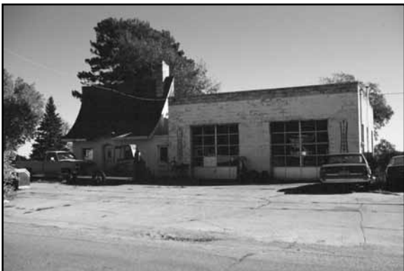
Gas station at southeast corner of Elm and South 3rd Street in Humphrey, PT05-079. House style gas station with service bays added demonstrating a transition of gas station form.
