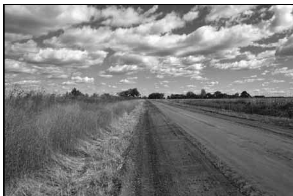
Current view of the Lincoln Highway in Lincoln County, LN06-239
