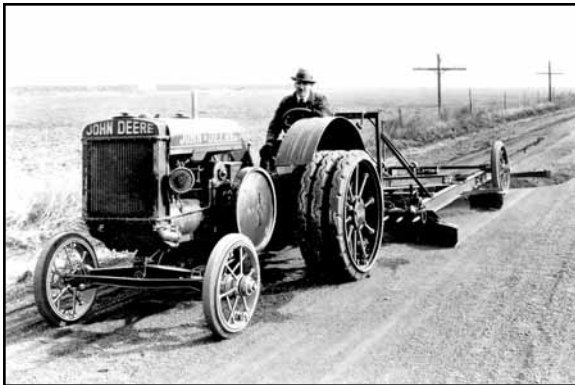
John Deere tractor pulling a road maintainer in an unknown rural location, 1920s-1930s (Photo courtesy of NDOR)
