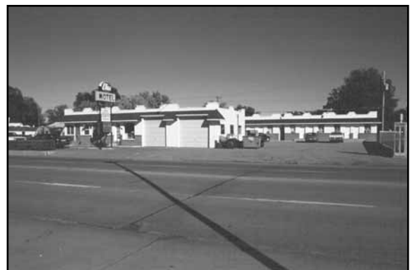
Elms Motel at the northeast corner of Highway 30 and G Street in Ogallala, KH04-122. Motel office building and lodging units.
