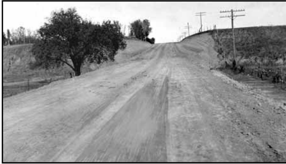
A "good dirt road" after construction on Highway 81 in Fillmore-Thayer Counties between Geneva and Belvidere in 1921 (Photo courtesy of NDOR)
