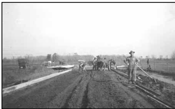
Laborers preparing subsoil for Highway 6 in Saunders County, c. 1921 (Photo courtesy of NDOR)
