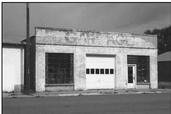
Commercial garage at the west side of Main Street, just north of Highway 30 in Brady, LN01-029.
