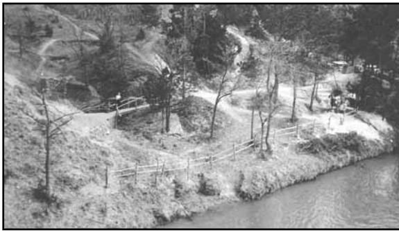
Roadside park on Niobrara River by the Bryan Bridge in Cherry County near Valentine in 1933 (Photo courtesy of NDOR)
