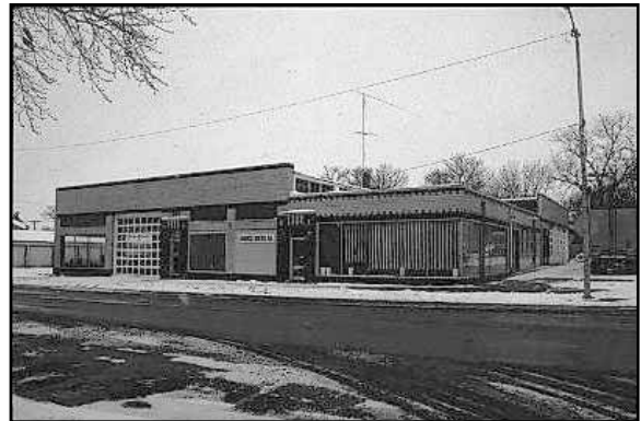
Voecks Motors Auto Dealership at the northeast corner of Main and 5th in Madison, MD03-086.
