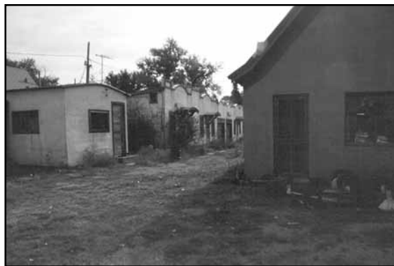
Motel, filling station and café at the northeast corner of Main and Highway 30 in Brady, LN01-030. Previously identified and recommended as potentially eligible.
