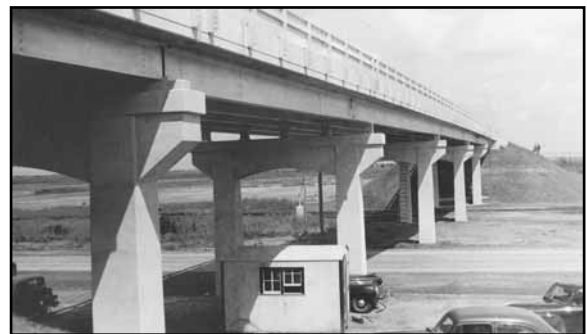
Overpass crossing between Highway 81 and Highway 6 in Fillmore County near Fairmont, 1941 (Photo courtesy of NDOR)
