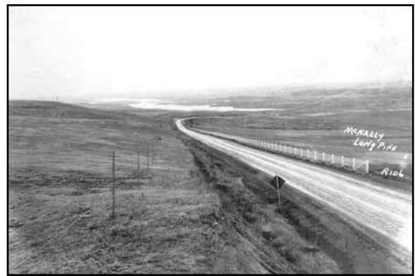
A completed portion of U.S. Highway 20 in 1927 in Brown County near Long Pine (Photo courtesy of NDOR)
