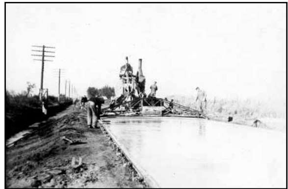
Paving 5.9 miles of the Lincoln Highway between Ames and Fremont in Dodge County, c.1920 (Photo courtesy of NDOR)
