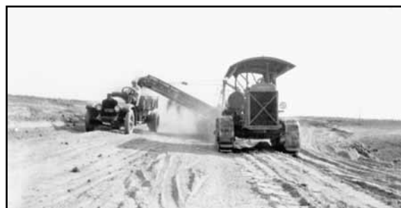
Dump truck being filled by an elevator in Phelps County, 1926 (Photo courtesy of NDOR)
