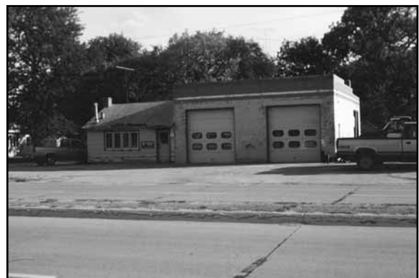
Service station at 419 Highway 6 in Holbrook, FN06-033. House form station with two-bay addition showing transition of gas station form.
