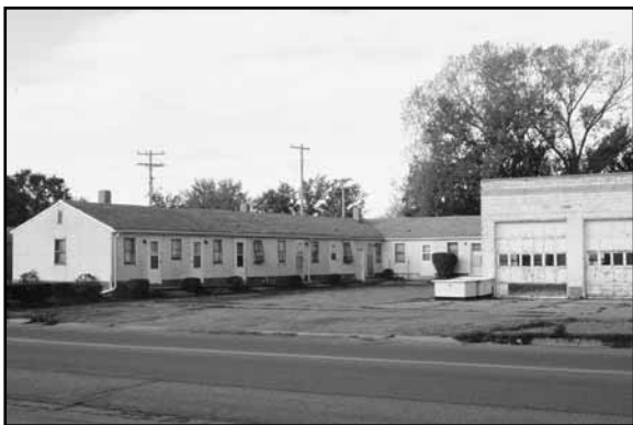
Motel court and service station at Main Street in Ainsworth, BW01-081
