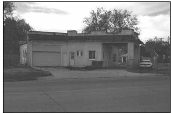
Service station at the southeast corner of B Street and Highway 30 in Schuyler, CX06-080. Service station features a central office with canopy and service bays extending on the sides.
