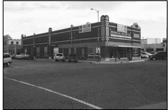
Reinecke Motor Company Garage at northeast corner of 11th and A Street in Schuyler, CX06-044. Two-story brick auto dealership.
