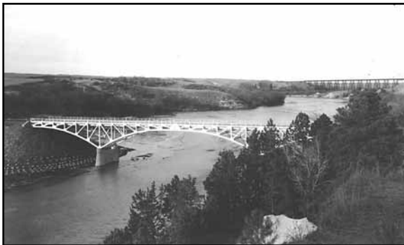
The Bryan Bridge shortly after its completion near Valentine, c. 1932 (Photo courtesy of NDOR)
