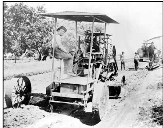
Cutting back slopes on the Lincoln Highway in Hall County, c. 1920 (Photo courtesy of NDOR)
