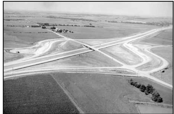
A county road crossing over I-80 in Cass County near Greenwood, 1961 (Photo courtesy of NDOR)
