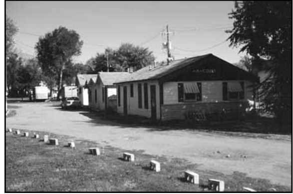
AA Motel at the northeast corner of 4 th Avenue and Sheridan Street in Holdrege, PP04-035. Motel court on the D-L-D.
