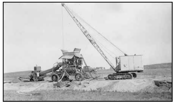
Oil and gravel mixer on U.S. Highway 20 in Cherry County near Thatcher in 1931 (Photo courtesy of NDOR)
