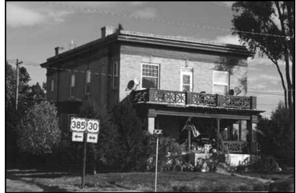
Hotel at 802 2nd Street in Chappell, DU02-060. Brick hotel probably originally constructed for the railroad.
