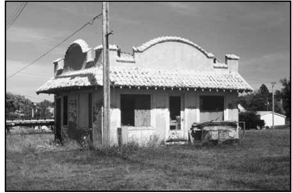
Spanish Colonial Revival style gas station south of Lincoln & 2nd Streets in Mullen, HO02-053
