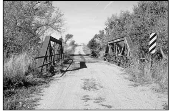
Pony truss bridge in Custer County near Ansley, CU00-084
