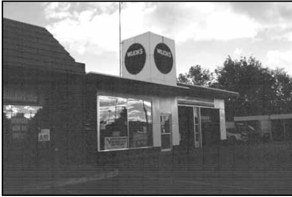
Service station at east side of Highway 81 between 7th and 8th Streets in Columbus (Also on the route of Meridian Highway), PT01-539. Porcelain enameled oblong box form gas station.
