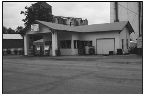
Belvidere Filling Station at 400 C Street in Belvidere, TY02-025. House style gas station with canopy constructed in 1925.
