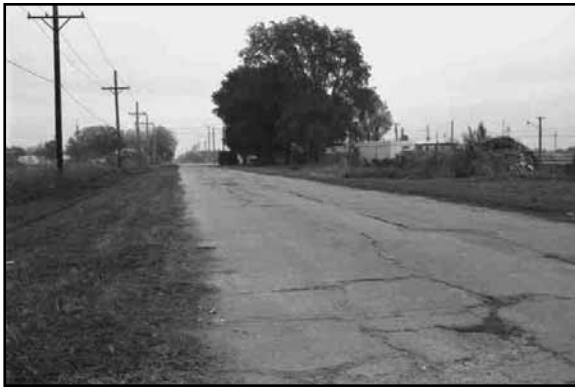
Seedling Mile at Seedling Mile Road between Willow and Stuhr Roads in Grand Island, HL06-696. One of the original concrete sections constructed to promote the use of hard paving along the highway. Previously determined eligible.
