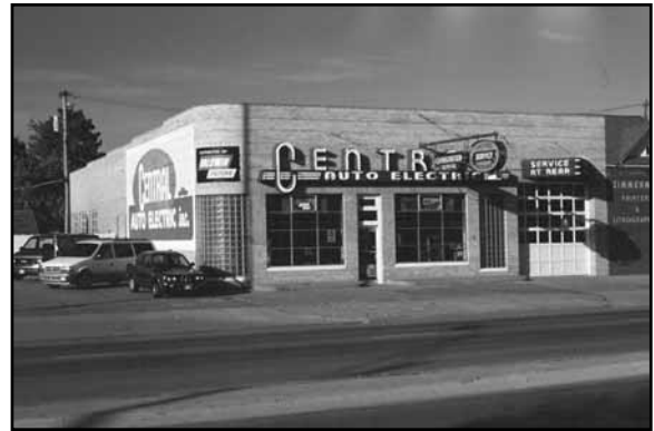
Central Auto Electric at north side 25th (Highway 30) between A Avenue and Central in Kearney, BF05-444. Streamline Moderne commercial garage with vintage neon signs.
