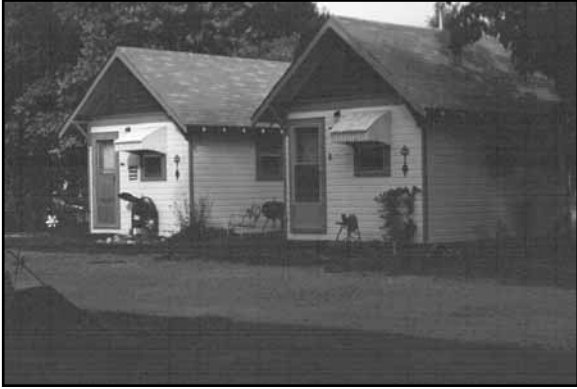
Arapahoe Cabin Court at north side of Chestnut between Nebraska and 7th in Arapahoe, FN01-070. Seven one-story, frame, front gable cabin units. Office is modern.
