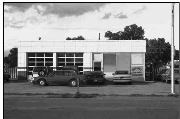
Service station at the northeast corner of 4th and McCabe Streets in North Platte, LN06-715. Oblong box form station with porcelain enameled steel panels.
