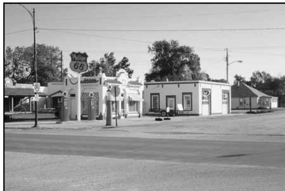
Spanish Colonial Revival style service station at the northeast corner of Clark & Legnard Streets in Bassett, R001-039
