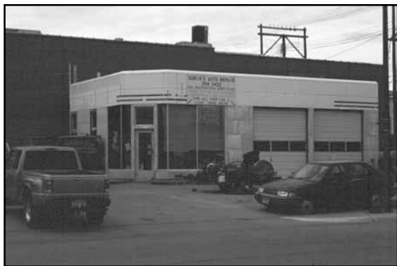
Service station at northwest corner of 9th Avenue and Illinois in Sidney, CN09-135. Porcelain enameled oblong box form gas station.
