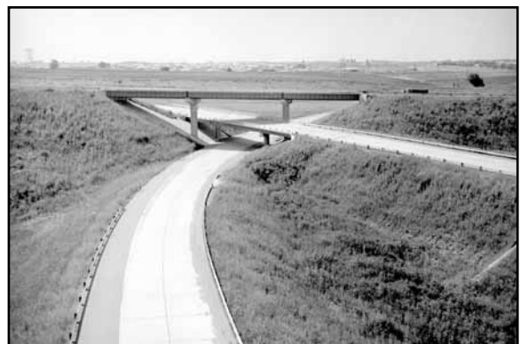
Tri-level overpass showing design standards for grade separation structures near Omaha, 1961 (Photo courtesy of NDOR)
