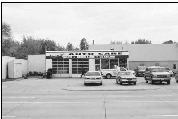
Service station at the southeast corner of Douglas & 5th Streets in O'Neill, HT13-146
