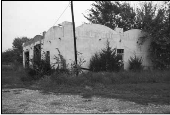
Hill Oil Terminal/Café at the northwest corner of Thompson and Highway 8 along abandoned curve of Highway 81 near Chester, TY00-257. Stucco service station and café designed in a southwestern style with projecting decorative roof beams extending through the wall. Also located on the route of the Potash Highway.
