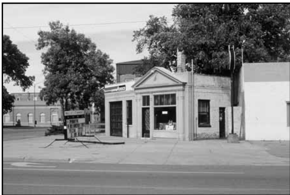
Neoclassical Revival style service station at the northeast corner of 10th & E Streets in Broken Bow, Custer County, CU05-072
