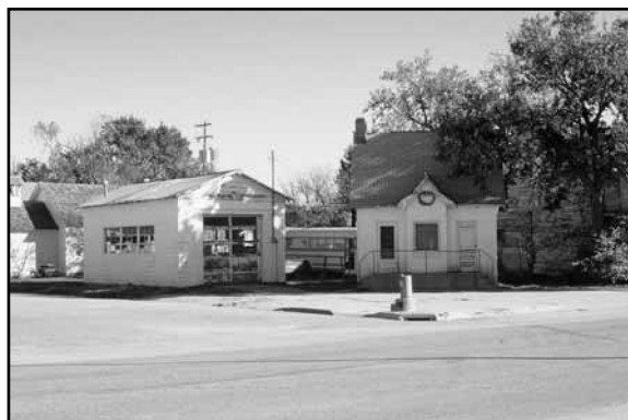
Service station at the northeast corner of Windom & 2nd Streets in Orchard, AP06-019
