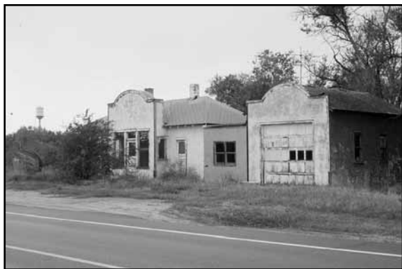
Service station by U.S. Highway 20 & Cherry Street in Cody, CE03-037
