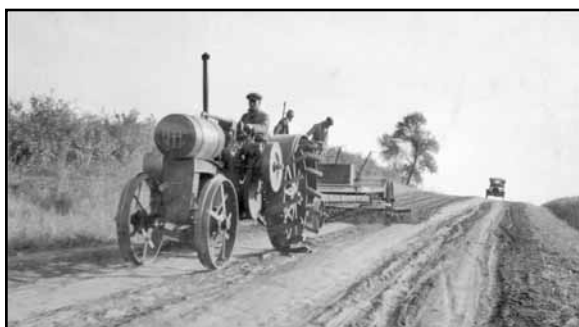
Example of a tractor pulling a road drag in order to grade the surface of a dirt road in Nebraska, location unknown, c. 1920s (Photo courtesy of NDOR)
