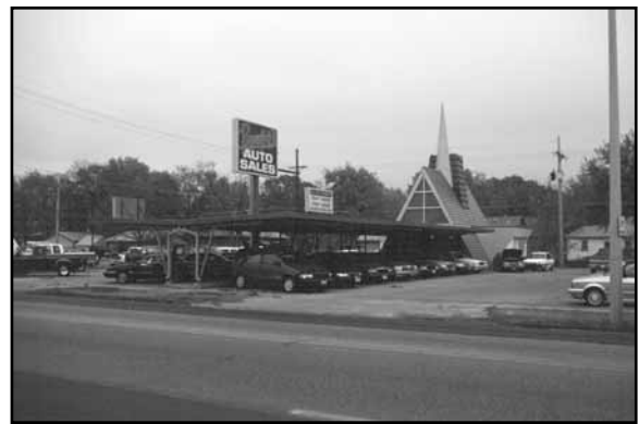
Drive-In at 1407 2nd Street in Grand Island, HL06-713
