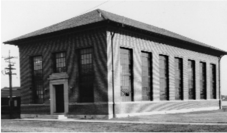
Building that housed the Atmospheric Wind Tunnel, the NACA's first wind tunnel (1920). Courtesy NASA Langley Research Center Photographic Archives.
