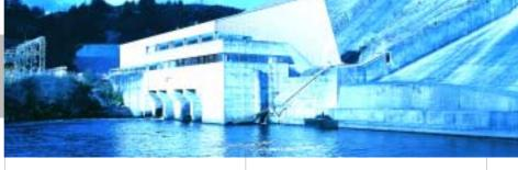
behind its 86 metre high dam, the Matahina scheme has two 36,000 kW generators producing an average annual output of 290 GWh. Significant maintenance work was completed on these machines during the decommissioning in 1997-98
