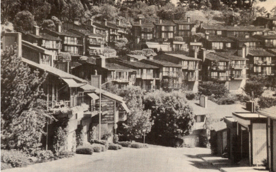
HILLER HIGHLANDS BEFORE
