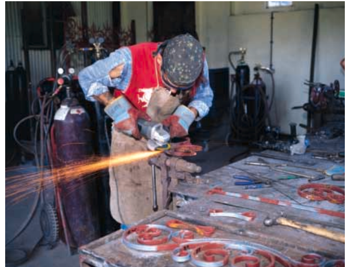
The Albert Memorial. Railings restoration work in progress at the workshop of Paul Dennis & Sons Ltd.
