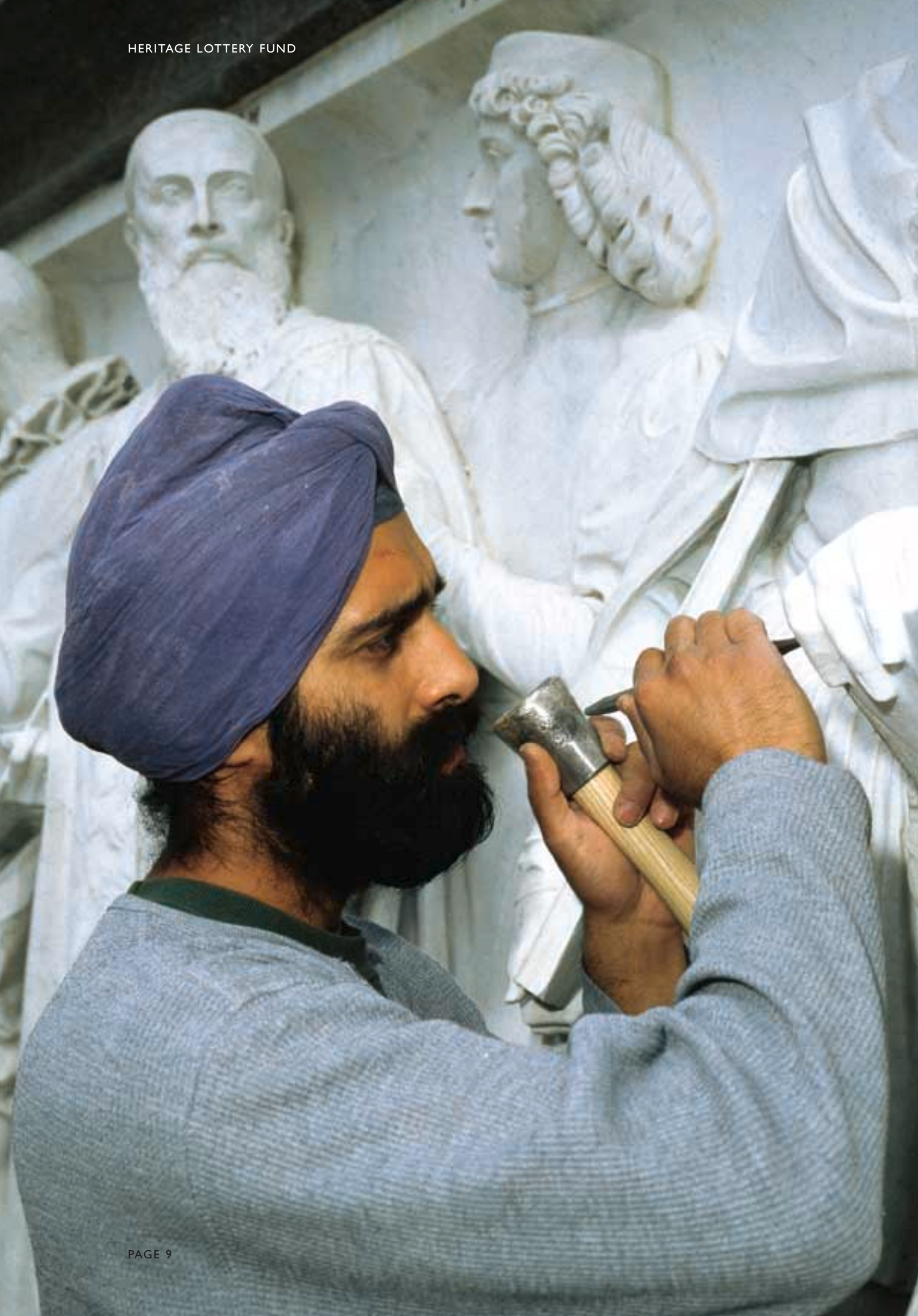
The Albert Memorial. Parnassus frieze restoration, work in progress.
