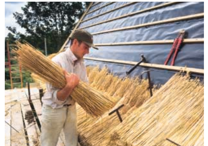
Thatching roof with combed wheat straw
