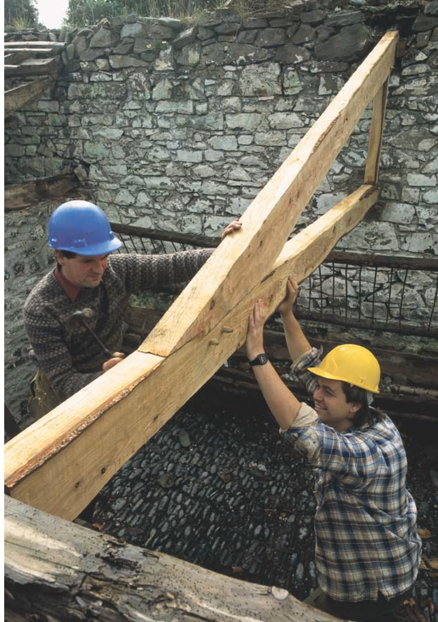
Conservationists propping up a wooden beam at Llanerchaeron.
