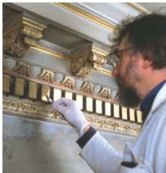
Broadsworth Hall. Plaster repair work in progress.
