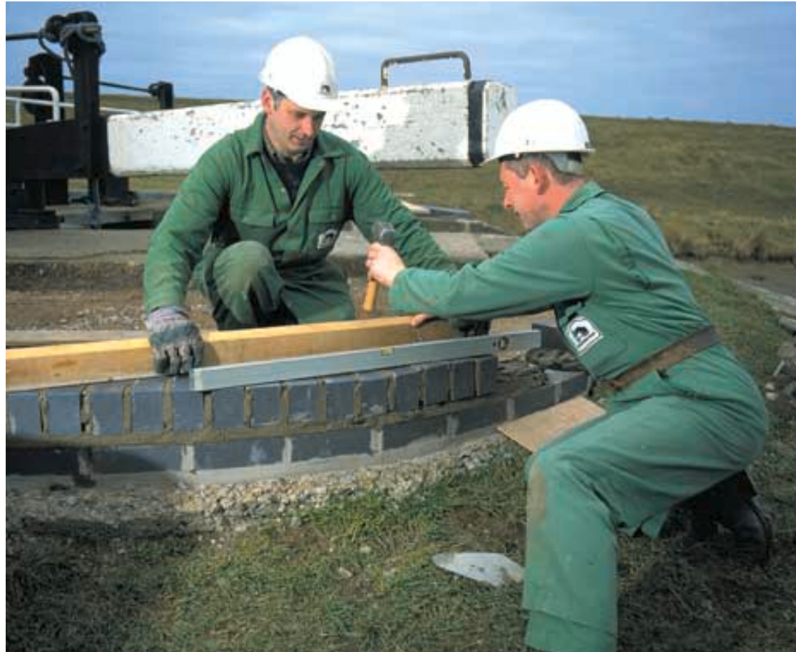
Lock restoration on Langollen Canal
