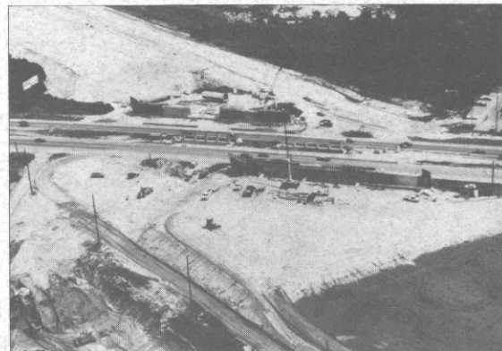
DelDOT is using recycled fly-ash (visible in lower right of photo) to construct the DAFB segment.
