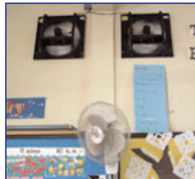
PV Fans cooling down a Nuuanu Elementary classroom (top two black colored fans side by side).
