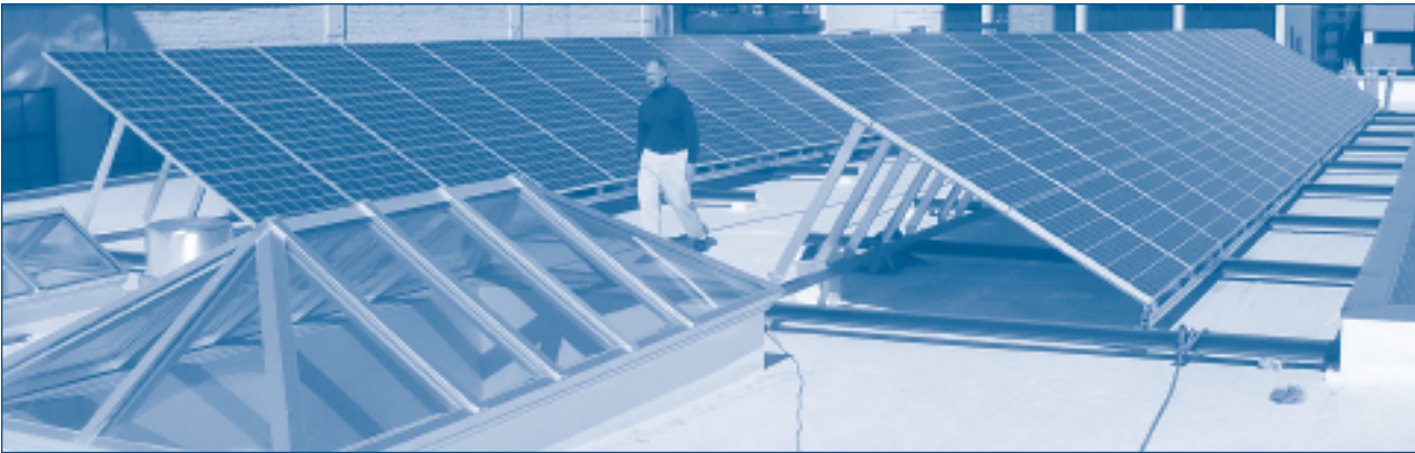
Rebuild America technical service provider Alan Nagle amid the solar panels atop the Acme building in Billings, MT.
