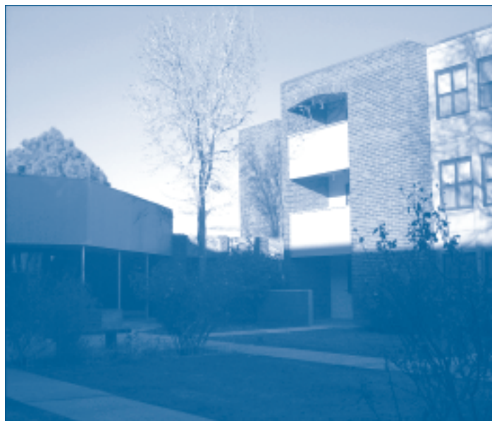
Wainwright Manor, above, a public housing complex in Albuquerque, will be retrofit for efficiency. The same will be done for Embudo Towers, below left.
