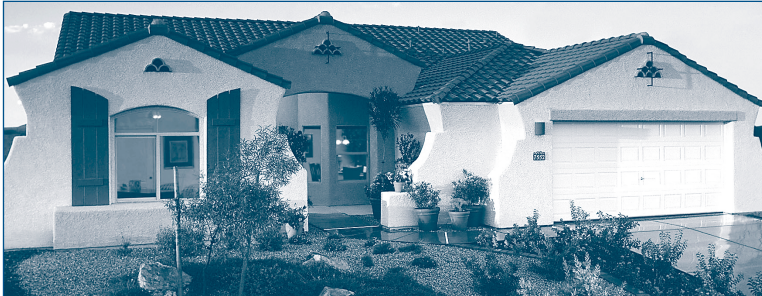
This cutting edge Pulte Home in Tucson, AZ, a collaborative effort of Building America's Building Science Consortium, was designed to reduce energy costs by as much as 50 percent.
