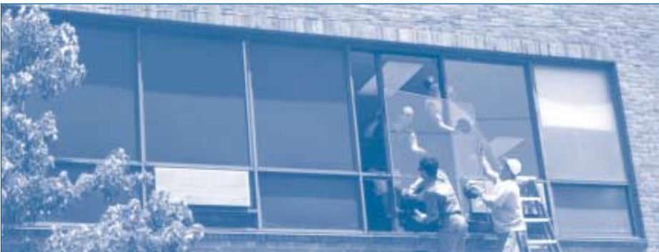
Window installers let the light in at Buist Academy.
