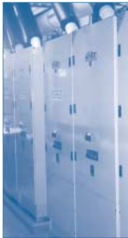
A boiler room in the newly renovated Kingston School District
