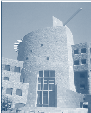
The Clark County Government Center, which houses 1,700 employees, is a showcase building of the county's energy conservation program.
