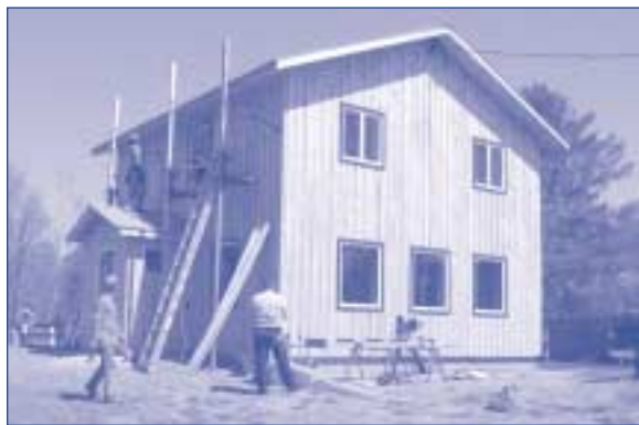
Habitat for Humanity house being built in Rensselaer Falls, NY.
