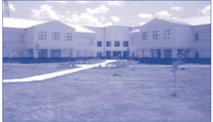
Hahnville High School in St. Charles Parish, LA, one of the Energy Fund project schools.
