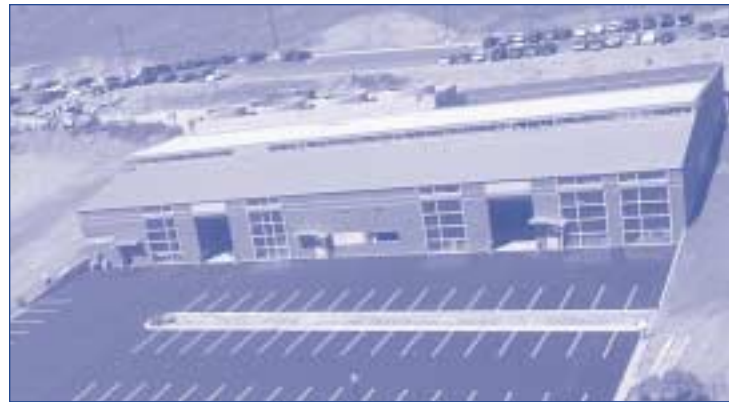
The new water plant at the University of Utah was an addition financed through guaranteed savings.
