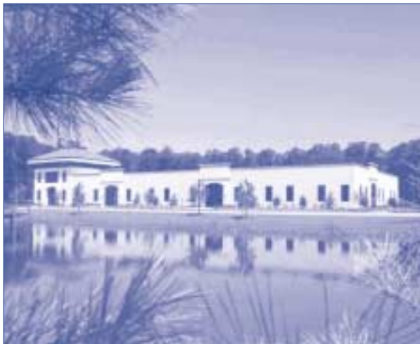
The Sustainable Technology Park building near Cape Charles harbor.
