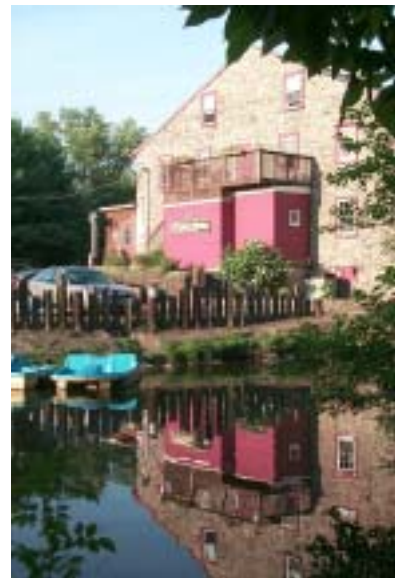
Fitzwater Station on Canal
