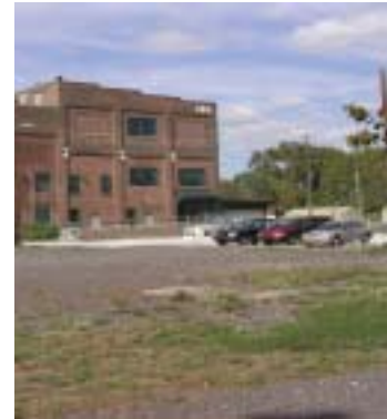
Old road at Trinley Mill
