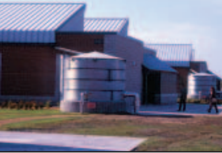
Using this cistern, the Roy Lee Walker Elementary School, in McKinney, TX, harvests rainwater.
