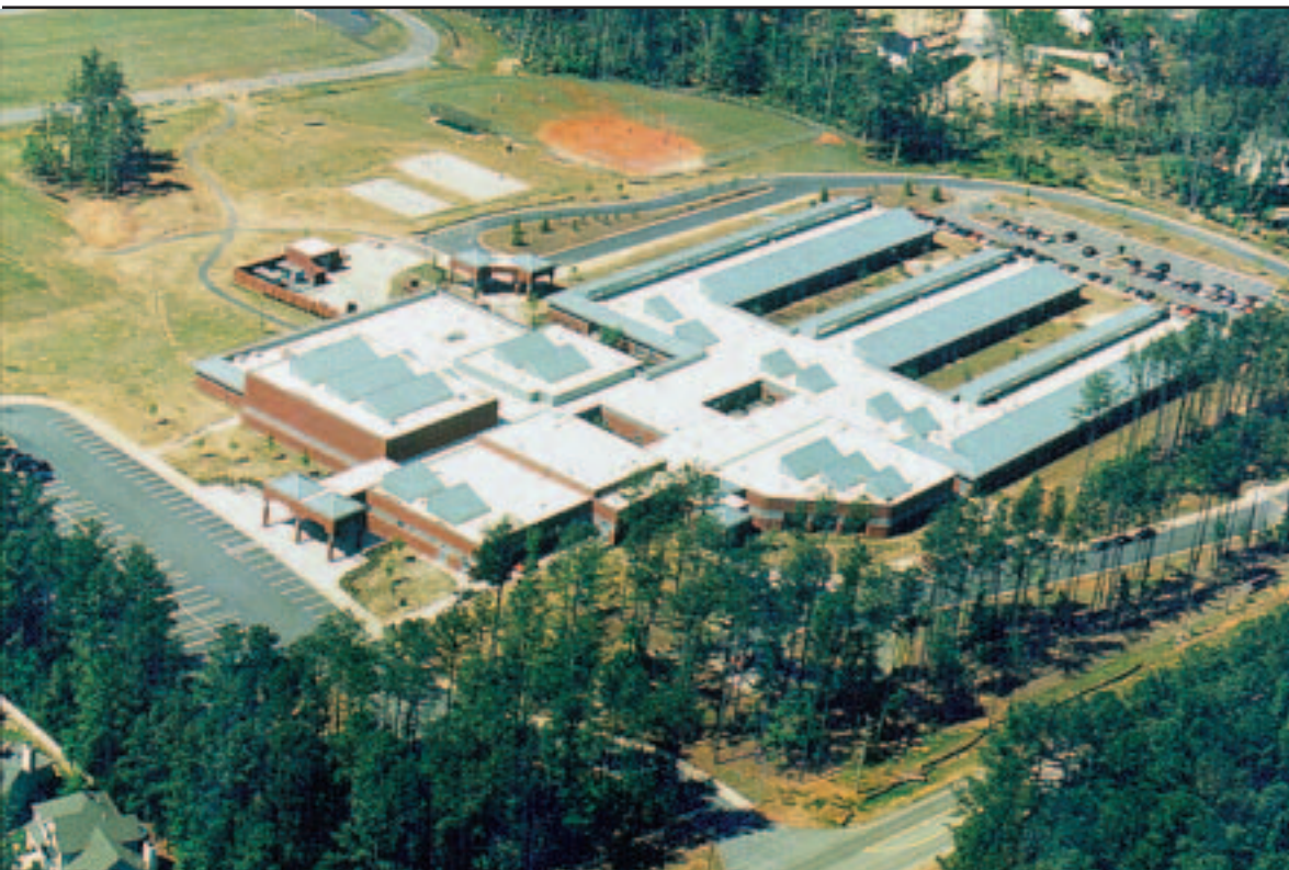
Durant Road Middle School in Raleigh, NC, is oriented on an east-west axis to maximize solar access.
