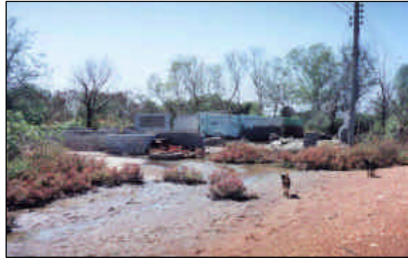
Remaining part of a farmhouse of an abandoned shrimp farm
