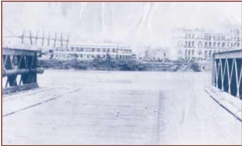
The 1893 demolition by flood of Victoria Bridge severed every type of engineering service: tram rails, water main, gas main and telephone (view from the south bank) [JOL negative 55983]
