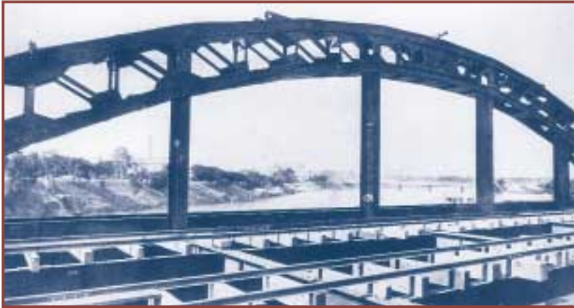
The 1897 Victoria Bridge and the recently completed City Hall seen through an arch of the Grey Street (later William Jolly) Bridge during construction in 1931 [JOL negative 63830]
