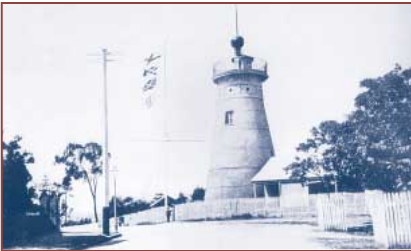
The 1828 Tower Mill observatory and signal station c. 1910: a telephone post, a gas street light and stone kerb and channel are evident in the left foreground [JOL negative 185525]
