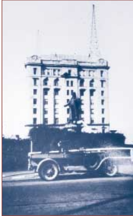
View from William Street across Queen's Park before May 1942, showing twin 4QG aerial support masts, each 30m high [JOL negative 185526]
