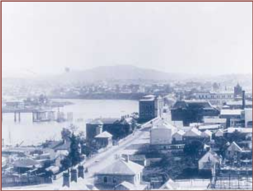
William Street c. 1873 viewed from Parliament House, showing the first permanent Victoria Bridge under construction, with Pettigrew's sawmill in the left foreground [JOL negative 163181]
