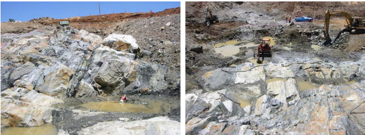
Figure 6: Wokalup Dam (2003) site showing the intense foliation and banding in the gneisses close to the Darling Fault.
