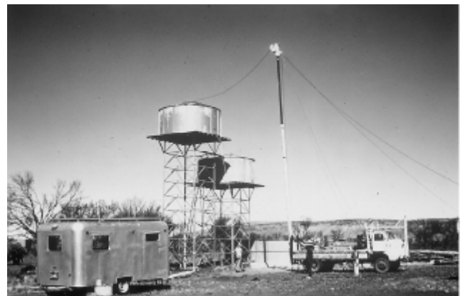
The Mines Department drilled for water in and around the North-West Aboriginal Reserve in 1970 and 1971 on behalf of the Department of Aboriginal Affairs. Four engine-driven and seven hand-operated pumps, four windmills and storage tanks were installed to provide water supplies for the Pitjantjatjara people. Being erected by the Department at Indulkana in 1971 were this 5000 gallon tank on a 30-foot stand and 48-foot windmill. (Photo T21773)
