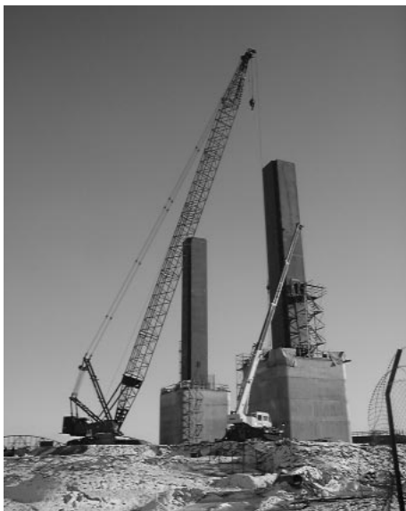
(a) Erection with 150 tf lifting crawler crane
