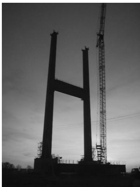
Fig. 12 Erection of main tower
