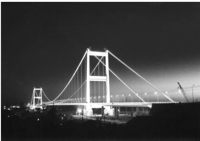
Fig. 1 “Irtysh River Bridge”
