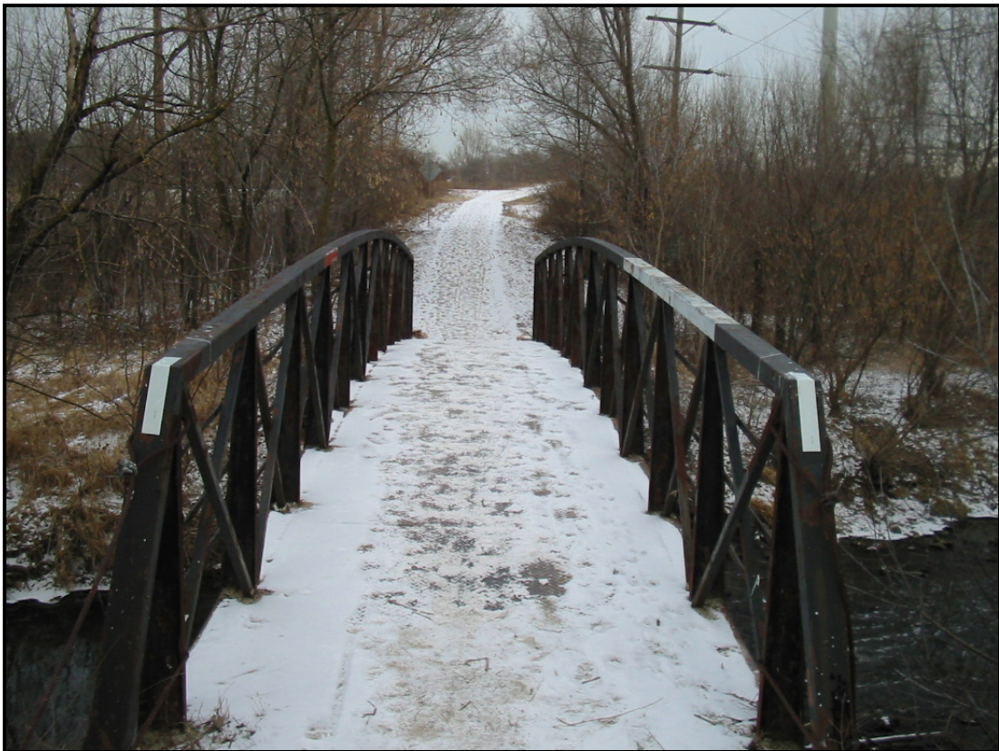
Existing Illinois Prairie Path Bridge Proposed for Replacement
