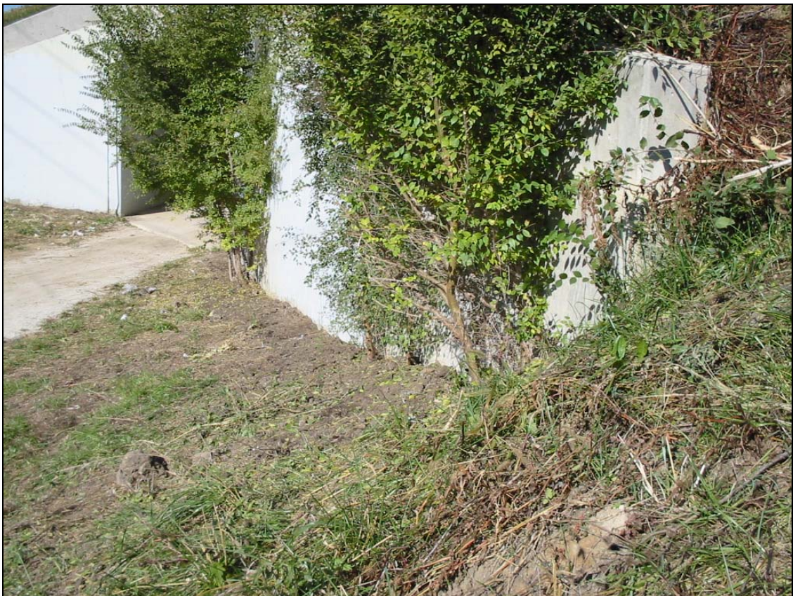
New Plantings Along Wing Walls at North Avenue Underpass
