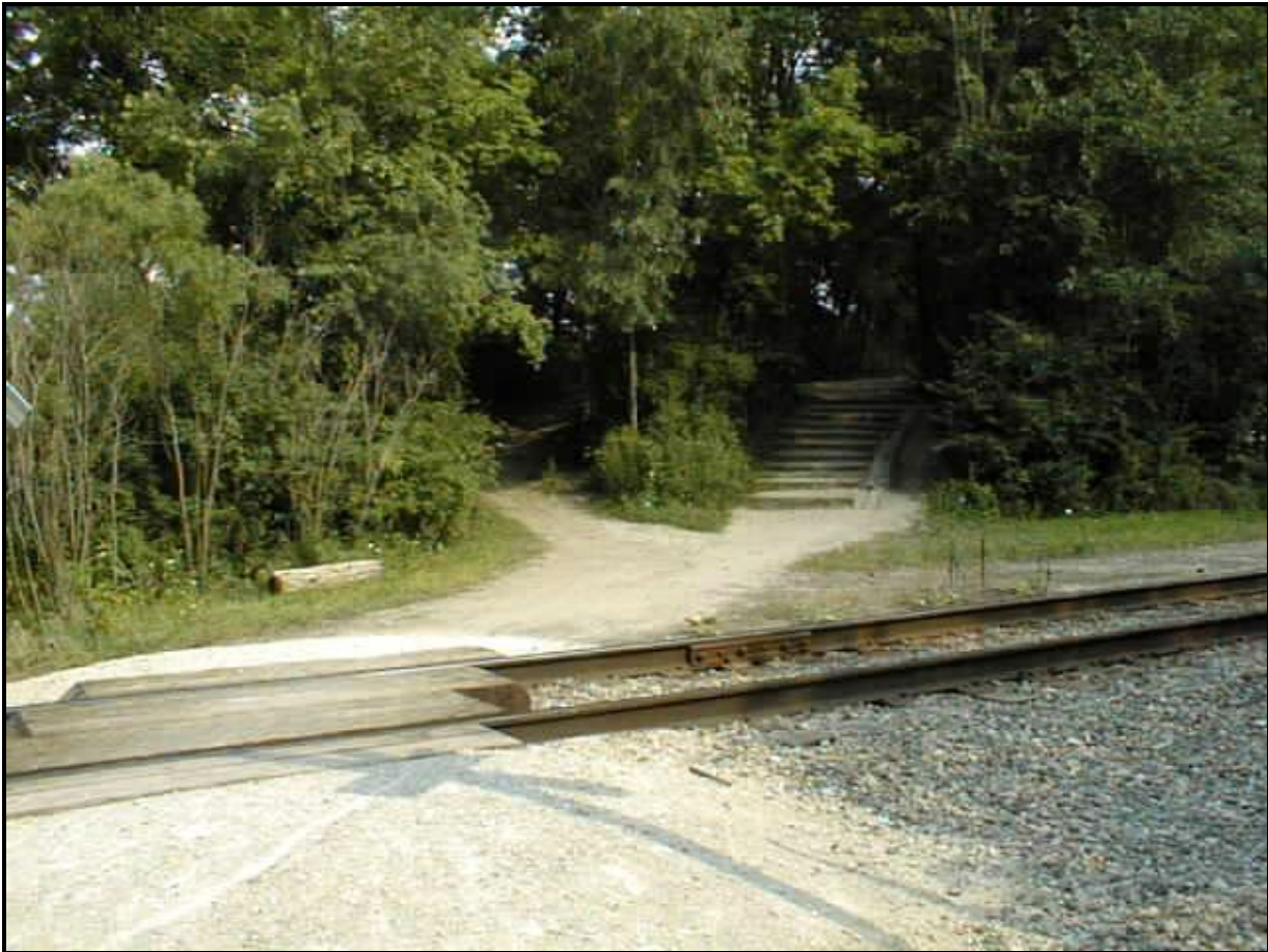
EJ&E Railroad Crossing along IPP Elgin Branch, Wayne
