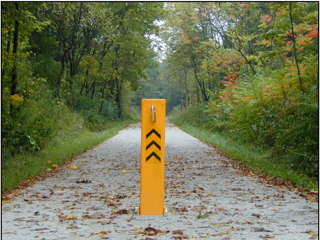
New Bollards Installed at 76 Locations Along the Trail System
