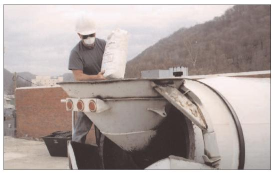
**FIGURE 7.6.** Adding repulpable bags of densified silica fume directly to truck mixer. See Section 7.3 for precautions regarding unopened bags. Note the use of a dust mask and safety glasses. See Chapter 9 for personal safety recommendations.
