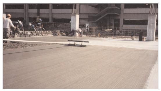
**FIGURE 8.17B.** This photo shows a finishing tool that is a combination of a float and a broom. In one direction, it serves as a float. In the other direction, it serves as a broom.
