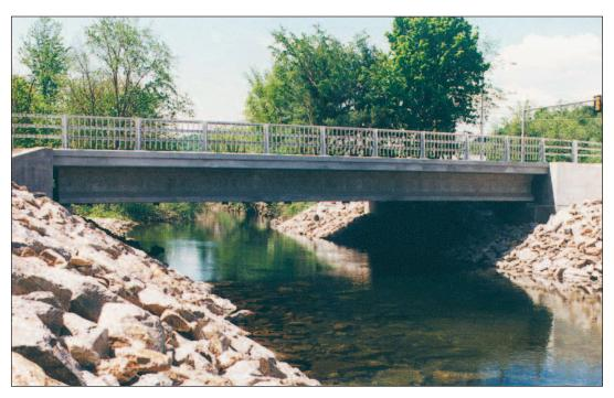
FIGURE 3.9. High-performance concrete bridge. In this bridge in New Hampshire, the high-strength concrete was used to reduce the number of girders required for the structure. For more information on this bridge, see the article by Wasczik (1999).
