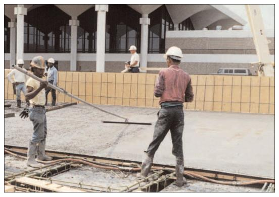
**FIGURE 8.16.** After screeding, the next finishing step is to bull float the concrete. Bull floating levels the surface and prepares the concrete to receive the texture desired.
