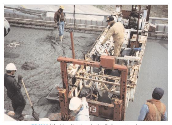
FIGURE 8.9. Bridge deck machine being used to place silica-fume concrete overlay.
