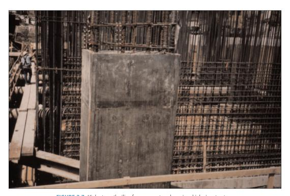
FIGURE 3.7. High-strength silica-fume concrete column in a high-rise structure.
