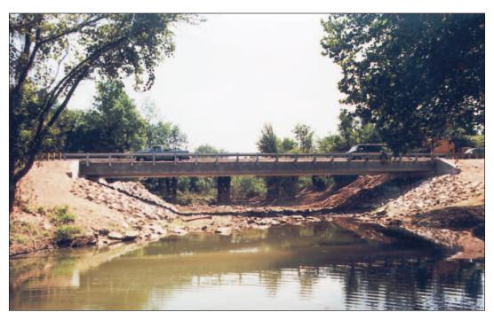
**FIGURE 3.8.** High-performance concrete bridge. In this bridge in Ohio, the high-strength concrete was used to increase span length and eliminate a pier in the river. For more information of this bridge, see the article by Miller (1999).
