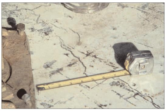
FIGURE 8.3. Plastic shrinkage cracks in silica-fume concrete.
