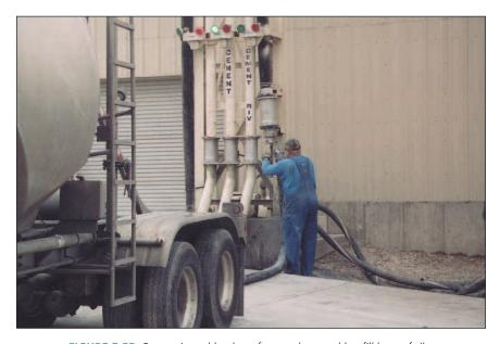
FIGURE 7.5B. Connecting rubber hose from tanker to rubber fill hose of silo.
