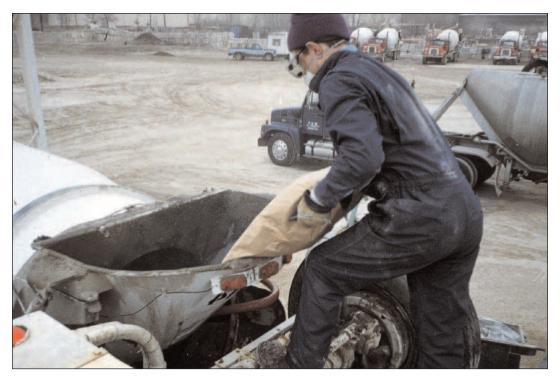
FIGURE 7.8. Emptying a bag of densified silica fume into a truck mixer.
