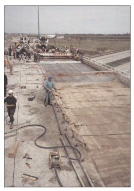
FIGURE 8.11B. Curing silica fume bridge deck. Note that curing is following placement and finishing without any delay.
