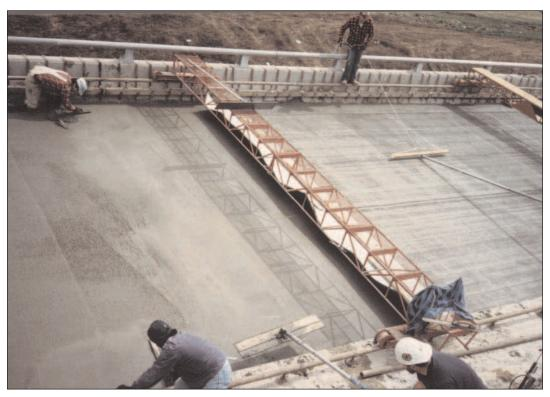
**FIGURE 8.10A.** Applying a broomed finish. After the finishing machine passes over the surface, some additional floating and finishing by hand may be required, particularly along the edges of the placement. Texturing using a broom can also be seen in this photo. State DOTs differ in their requirements for texturing of bridge decks — some require brooming, some tining, and some require that the texture be sawn into the concrete after hardening.
