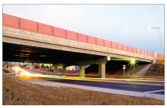
**FIGURE 3.10.** High-performance concrete bridge. In this bridge in Colorado, the high-strength concrete was used to increase span length to eliminate two piers and to increase the head room under the bridge. For more information on this bridge, see the article by Leonard (1999).
