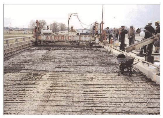
**FIGURE 8.7.** Concrete bridge deck prepared for a silica-fume concrete overlay. Deteriorated concrete has been removed and the reinforcing steel has been cleaned to prepare for the placement of the overlay.
