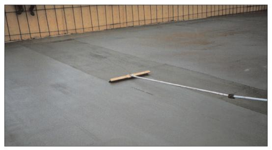
**FIGURE 8.17C.** Brooming of a silica-fume concrete surface. In this case, the broom has a wire attached to it to lift it off the surface for travel from right to left in the photo. The texture is applied by pulling the broom from left to right.
