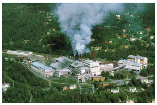
**FIGURE 1.2.** Smelter before installation of equipment to collect silica fume. The "smoke" is silica fume being released to the atmosphere. Today, in the U.S., no silica fume is released — it is all captured and used.
