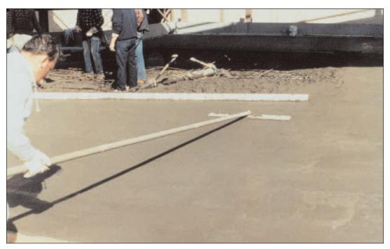
**FIGURE 8.17A.** Depending upon the nature of the surface finish selected, it may be necessary to perform one additional pass with a float before the surface texture is applied.
