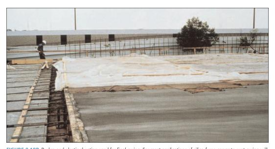
**FIGURE 8.18B.** Burlap and plastic sheeting used for final curing. For most applications of silica-fume concrete, wet curing will provide better in-place concrete quality than the use of curing compound alone.
