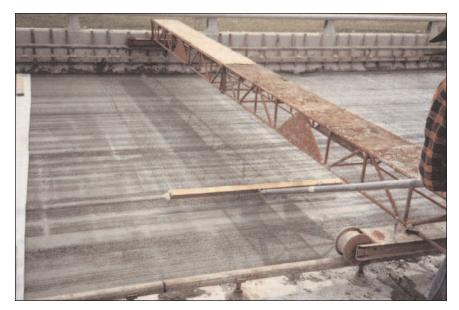
**FIGURE 8.10B.** Applying a tined finish. Note that some DOTs prefer to have the grooves ground in after the concrete has hardened.
