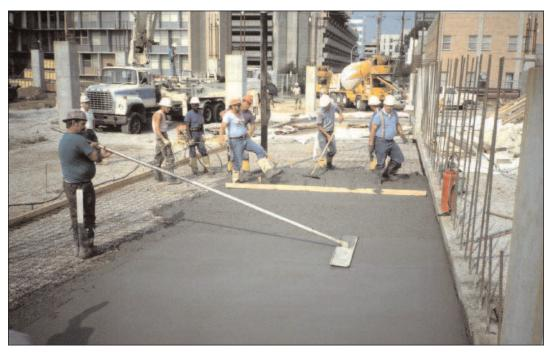
**FIGURE 8.14.** Conducting a trial placement using the one-step finishing procedure. Note that the trial is a slab on ground on the actual structure. Note that placing the wire mesh on the bottom of the slab is not recommended practice.
