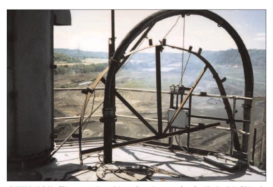
FIGURE 7.4C. Rubber fill hose connected to steel pipe on silo top. Note support frame for rubber hose being fabricated.
