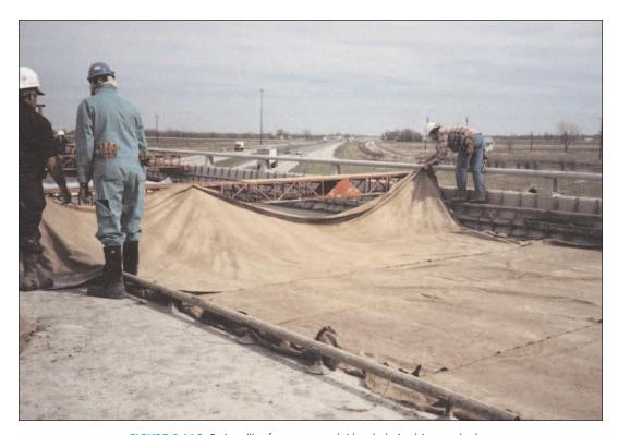
FIGURE 8.11C. Curing silica-fume concrete bridge deck. Applying wet burlap.
