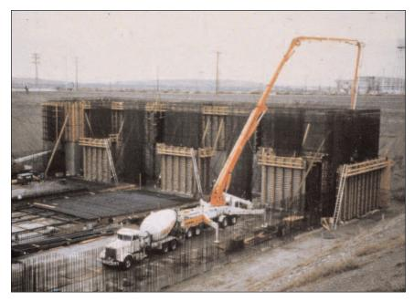
**FIGURE 3.16.** Concrete containing portland cement, fly ash, and silica fume being placed. The fly ash was used to control heat of hydration while the silica fume provided early strength required for stripping forms. For more information on this project, see the article by Holland (1998).
