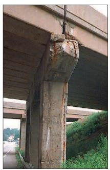
**FIGURE 3.14.** Chloride induced corrosion on a highway overpass. Note that chlorides have apparently run off of deck and onto this pier. Structural elements as well as decks should be protected.
