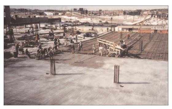
**FIGURE 3.4.** "One-pass finishing" of silica-fume concrete in a parking structure. Placing, finishing, texturing, and curing are done as a continuous process.
