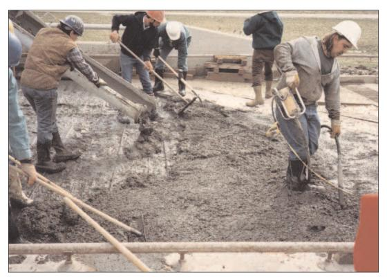
**FIGURE 8.8.** Silica-fume concrete being placed on the deck. Note the use of the vibrator to provide additional consolidation to that provided by the finishing machine.
