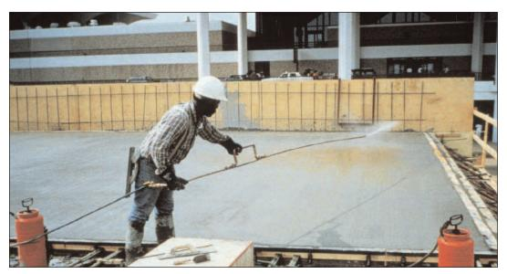
**FIGURE 8.18A.** Curing compound is being applied to silica-fume concrete in a parking structure shortly after brooming. In many cases, the use of curing compound is the preliminary curing method; it is intended to protect the concrete until it gains enough strength to allow placing wet curing materials on the deck without marring the surface. On this particular project, wet burlap and plastic sheeting were used for the final curing.
