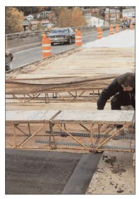
FIGURE 8.11A. Wet curing using burlap and plastic sheeting applied to a silica-fume concrete bridge deck.
