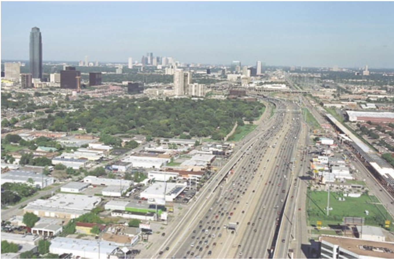
Houston's busiest freeway: The Southwest Freeway just outside Loop 610 is Houston's busiest freeway, with 337,000 vehicles per day in 2001. The reconstruction to its present configuration with 12 main freeway lanes was completed in 1992. At the right side of this photo, construction on the Westpark Tollway, an elevated structure at this location, is in progress. (Photo: September 2002)
