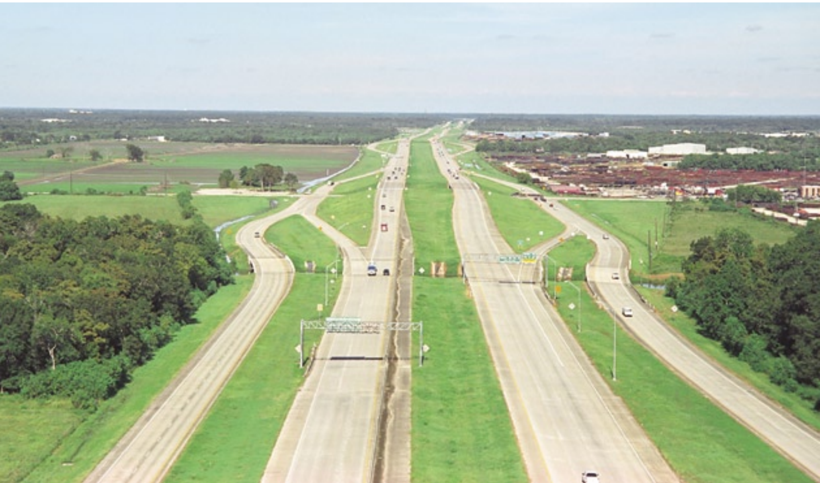
Crosby Freeway: This view looks east along the semi-rural freeway. (Photo: September 2002)
