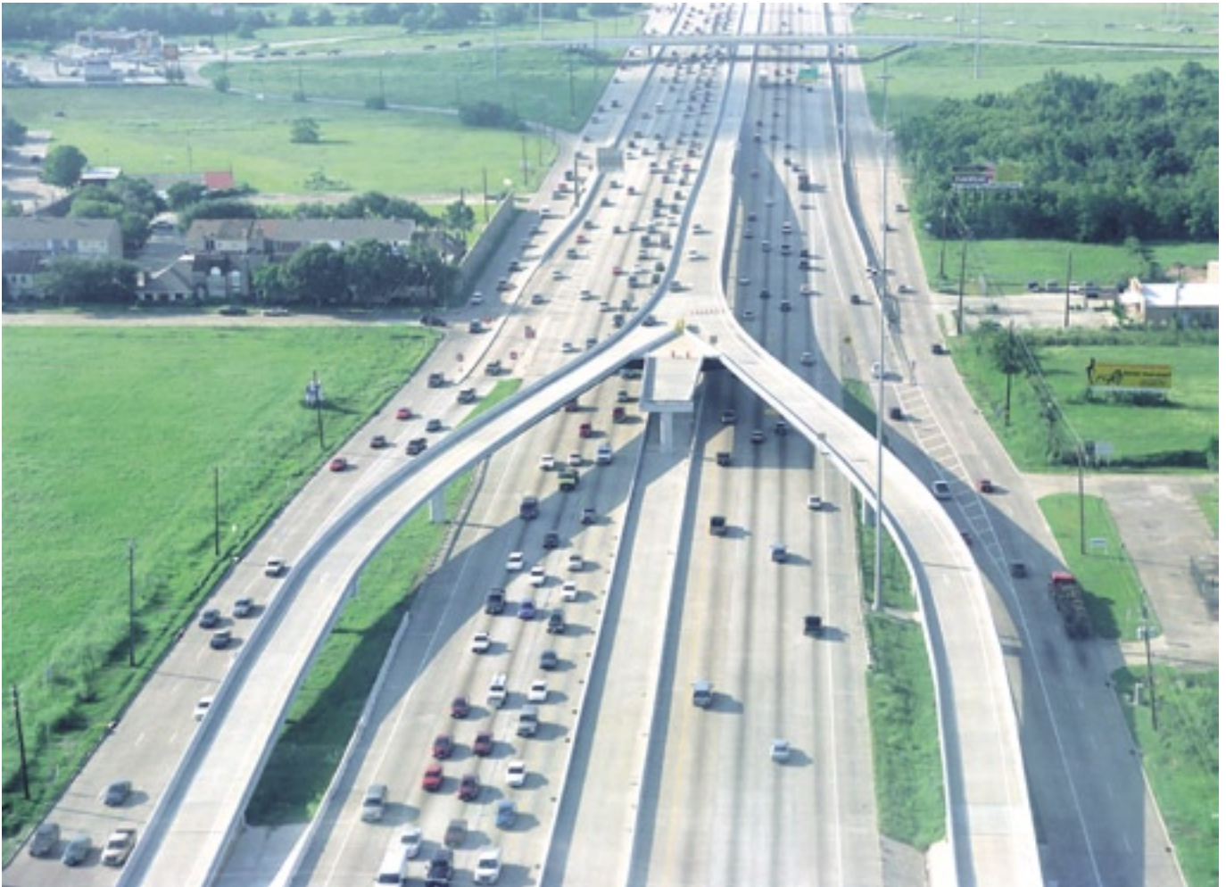
The Gulf Freeway wishbone: This transitway access structure was completed in 1997 just south of Beltway 8. (Photo: James Lyle, TTI, June 2001)
