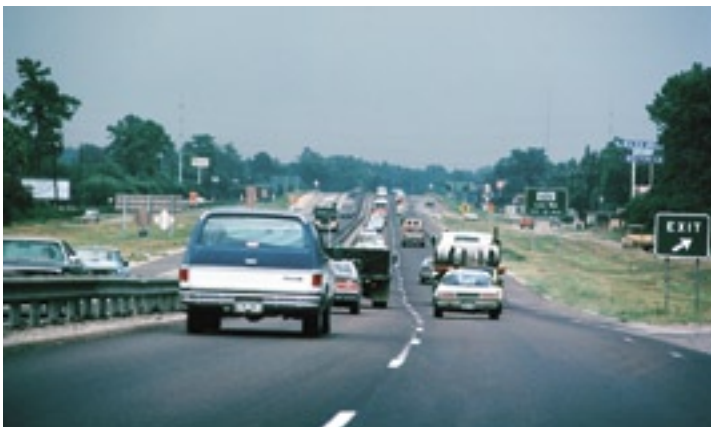
Original Eastex: This view dated August 1981 shows the original four-lane freeway just north of Aldine Mail Road. Expansion of this section was completed in 1998. (Photo: Texas Transportation Institute)
