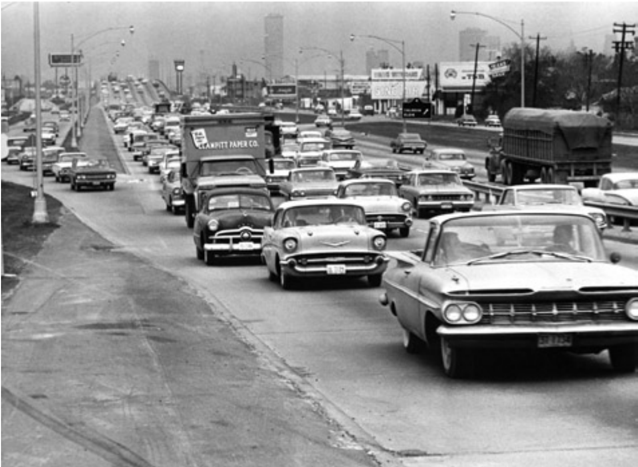
Ramping up to danger: This 1963 photo illustrates design and safety hazards in the original Gulf Freeway. The freeway on-ramp has practically no merging space and was the most accident-prone spot in Houston in 1963. Also shown is a row of light fixtures positioned within about 12 feet (3.7 m) of the main traffic lanes. Breakaway fixtures had not yet been developed in 1963, and these obstructions were a serious hazard to motorists. 13 (Photo: Houston Chronicle )
