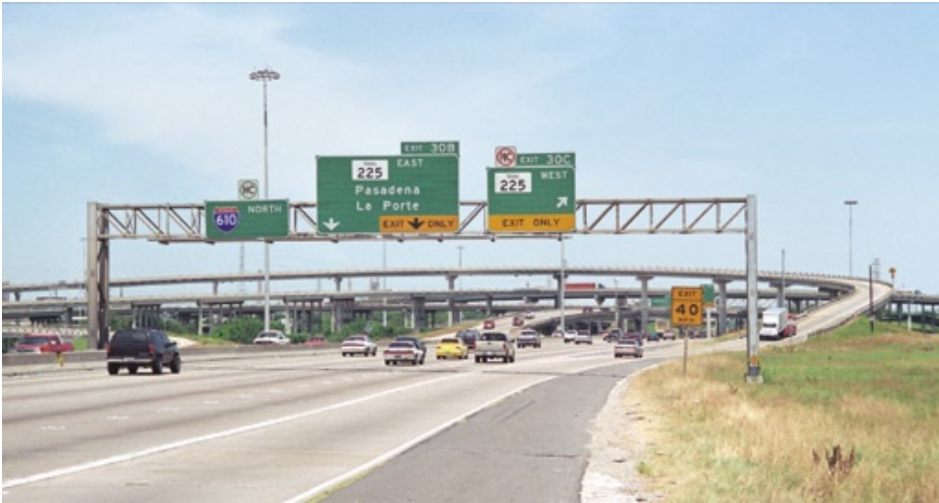
Ramp to a dead end: This view along Loop 610 at the SH 225 interchange shows the exit and high-level connection ramp to SH 225 west, the planned Harrisburg Freeway. The freeway comes to a dead end just after the ramp returns back to ground level. (Photo: May 2002)
