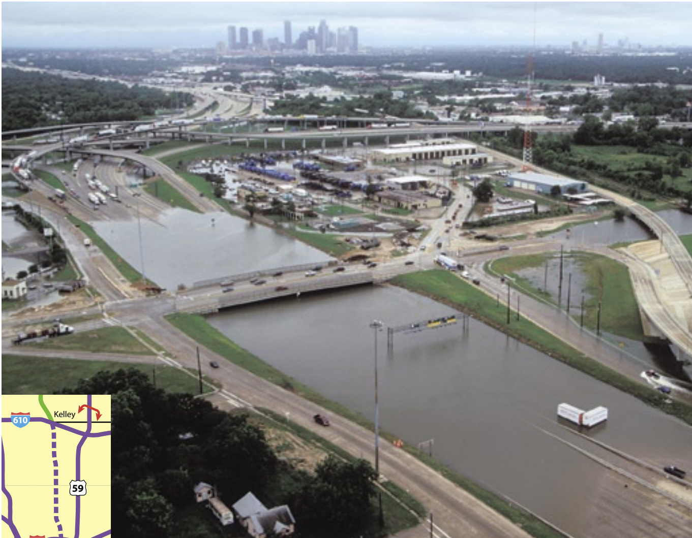
Tropical Storm Allison: The storm unleashed a huge flood event on Houston in June 2001. The Eastex Freeway drops below ground level at only one point. As shown above, the underpass was completely filled with water. (Photo: copyright Jim Olive/Stockyard.com)
