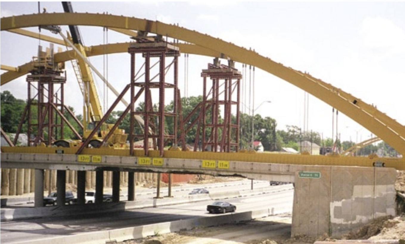
Houston's most appropriately named street: For 40 years Hazard Street was, in fact, one of Houston's most hazardous streets. The Hazard Street bridge over the Southwest Freeway had a clearance of only 13 feet, 11 inches (4.24 m) and was frequently the scene of collisions with oversize vehicles. The damage to the bridge structure (underneath the height signs) visible in the photo was not part of the demolition process—it was the result of collisions during the previous 40 years. The replacement span is an arched structure with improved vertical clearance. On August 12, 2000, the original bridge was demolished. (Photo: Chuck Fuhs)
