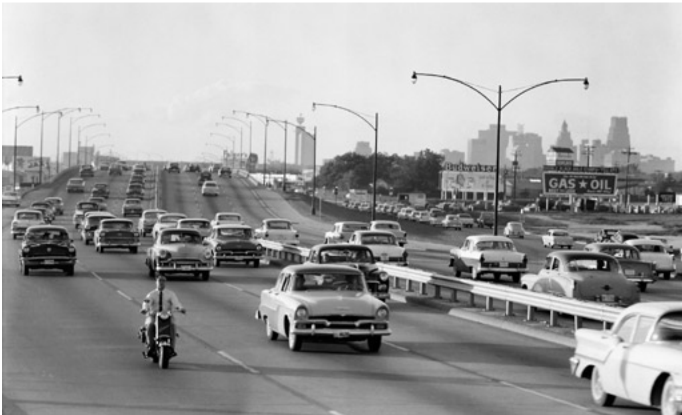
Crossing over to safety: The most serious design flaw of the original Gulf Freeway was the lack of a center guardrail. The upper left photo shows a typical section of the original freeway with its curbed median. Prior to the installation of the barrier, there were 60 crossover accidents, resulting in 9 fatalities and 70 injuries. The upper right photo shows the installation of the median guardrail in 1956. The lower photo shows the freeway in the late 1950s. In the three years after the guardrail installation, there were no crossover accidents. (Photos: TxDOT)
