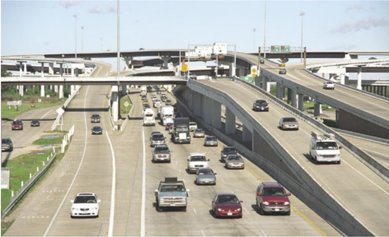
Northwest Freeway-Beltway 8 interchange: Although the Northwest Freeway itself is not impressive, the huge interchange at Beltway 8 is one of Houston's most impressive stack interchanges. The interchange was completed in 1990. This view looks northwest along the Northwest Freeway. The ramp in the center of the freeway (with the van and two vehicles) provides access to the transitway and is not part of the interchange. (Photo: March 2003)
