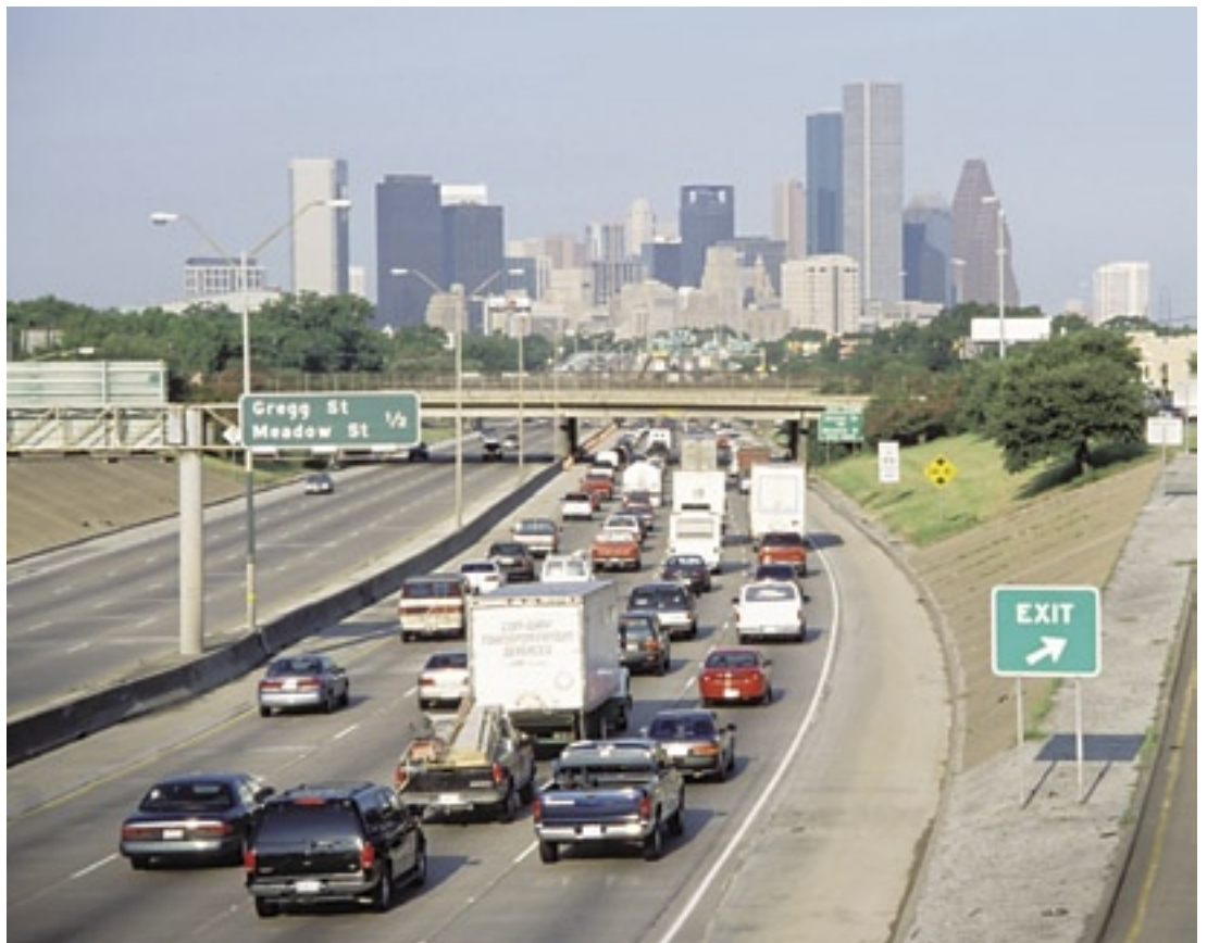
Downtown approach: This view looks west with the Waco Street overpass just ahead. (Photo: July 2002)
