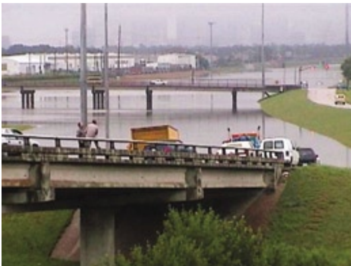
Lake 288: This view shows the South Freeway after Tropical Storm Allison in June 2001. In its early years the South Freeway was susceptible to flooding caused by water from Brays Bayou backing up into the freeway drainage system. Modifications to the drainage system and more powerful pumps alleviated most flooding but were not enough to prevent flooding during Allison. (Photo: Jonathan Miller)
