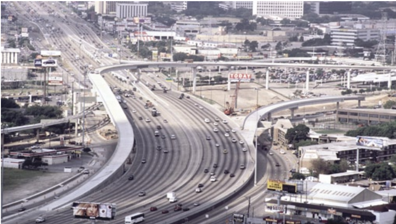
Southwest Freeway interchange: This view looks southbound along the Southwest Freeway (US 59), showing the connector ramps to the Westpark Tollway. The Westpark Tollway is in a trench at this point and is not visible in this view. (Photo: © Scott Teven/www.HoustonPhoto.com, May 2003)
