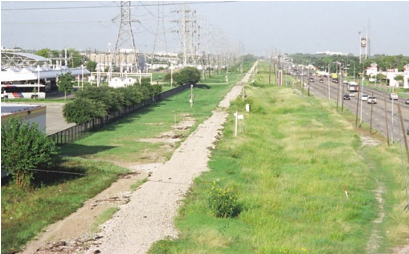
Pre-tollway Westpark: The above view looks west along the Westpark Drive corridor from the Southwest Freeway overpass in July 2001, just before tollway construction began. The Harris County Toll Road Authority acquired 50 feet (15 m) of the 100-foot (30 m) railroad corridor, roughly the section between the railroad bed and Westpark Drive on the right. The left views show the corridor before the railroad tracks were removed, with the upper view looking east at Beltway 8 and the lower view looking east at Old Westheimer Road. (Photos: upper, July 2001; left, November 2000)
