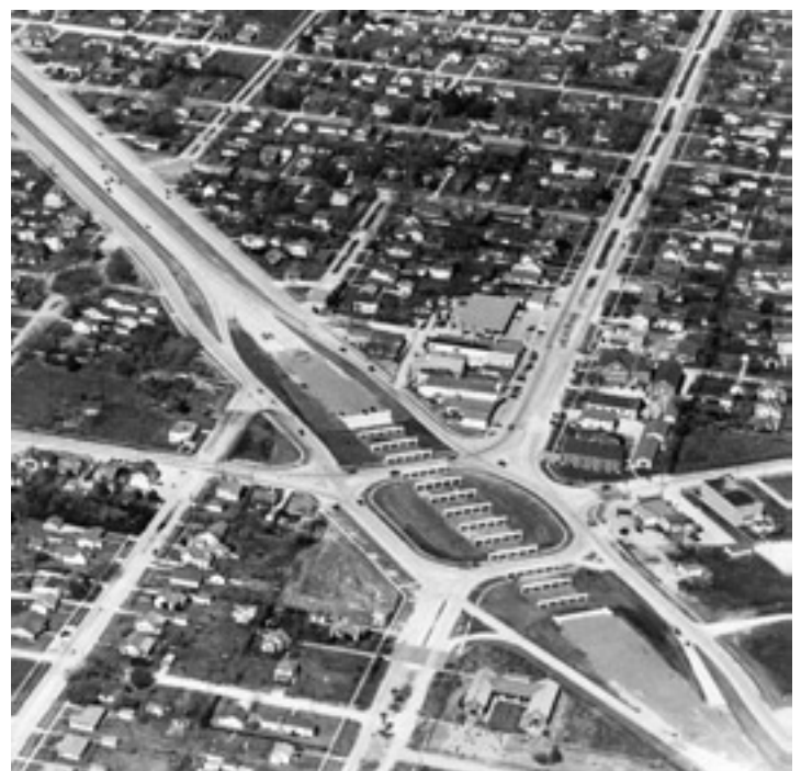
A Houston rarity: This view looks north at the Broadway intersection in early 1952. The intersection design included a traffic circle, and the same basic design remains in service in 2003. It is the only remaining traffic circle on Houston’s freeway system. (Photo: Greater Houston Partnership)
