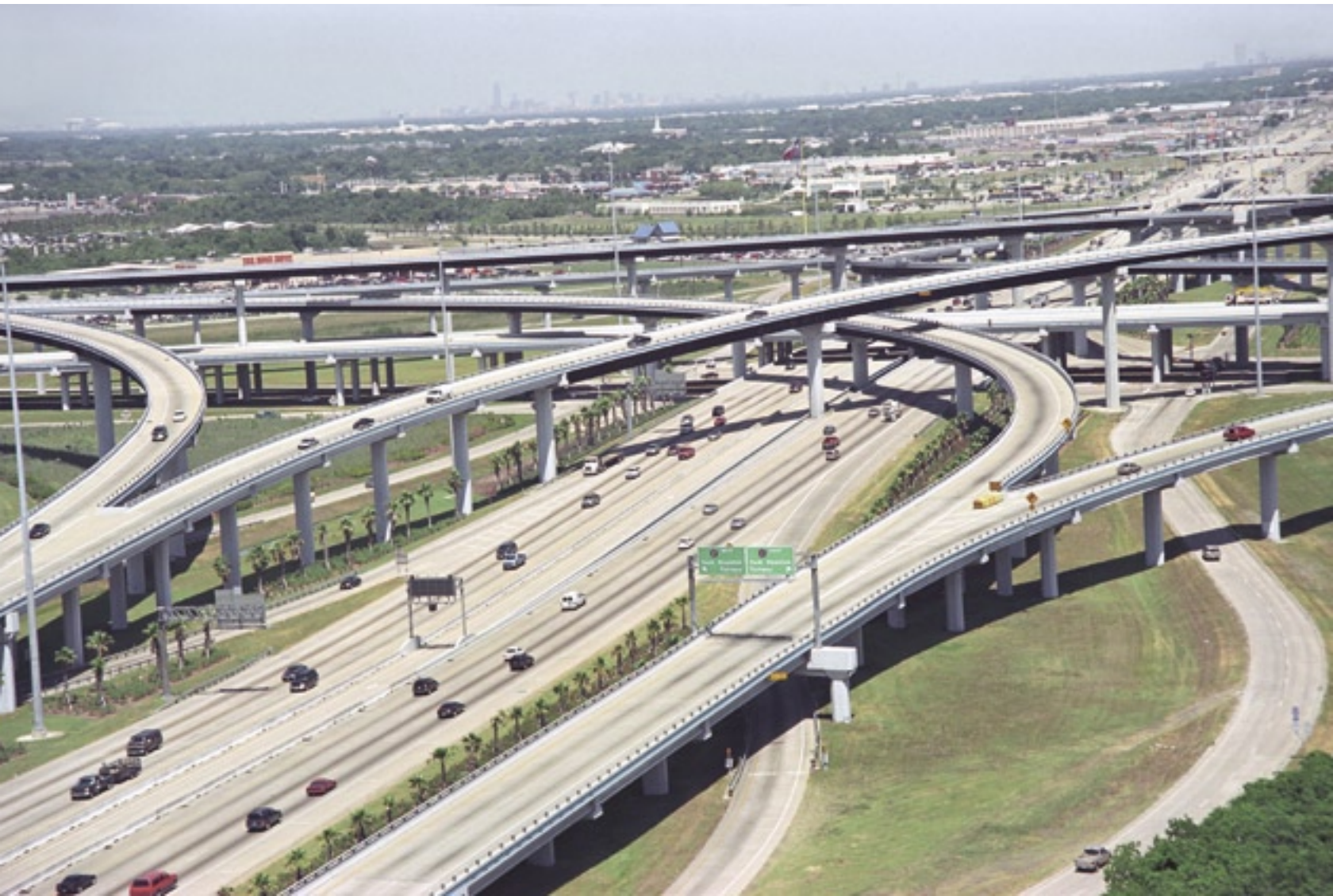
The ultimate stack interchange? The impressive interchange at the Gulf Freeway and Beltway 8 features high-flying ramps, symmetric design, and a sprawling right-of-way. This view looks northwest along the freeway. The completion of the interchange in 1997 capped 50 years of nearly nonstop construction on the Gulf Freeway. (Photo: May 2002)
