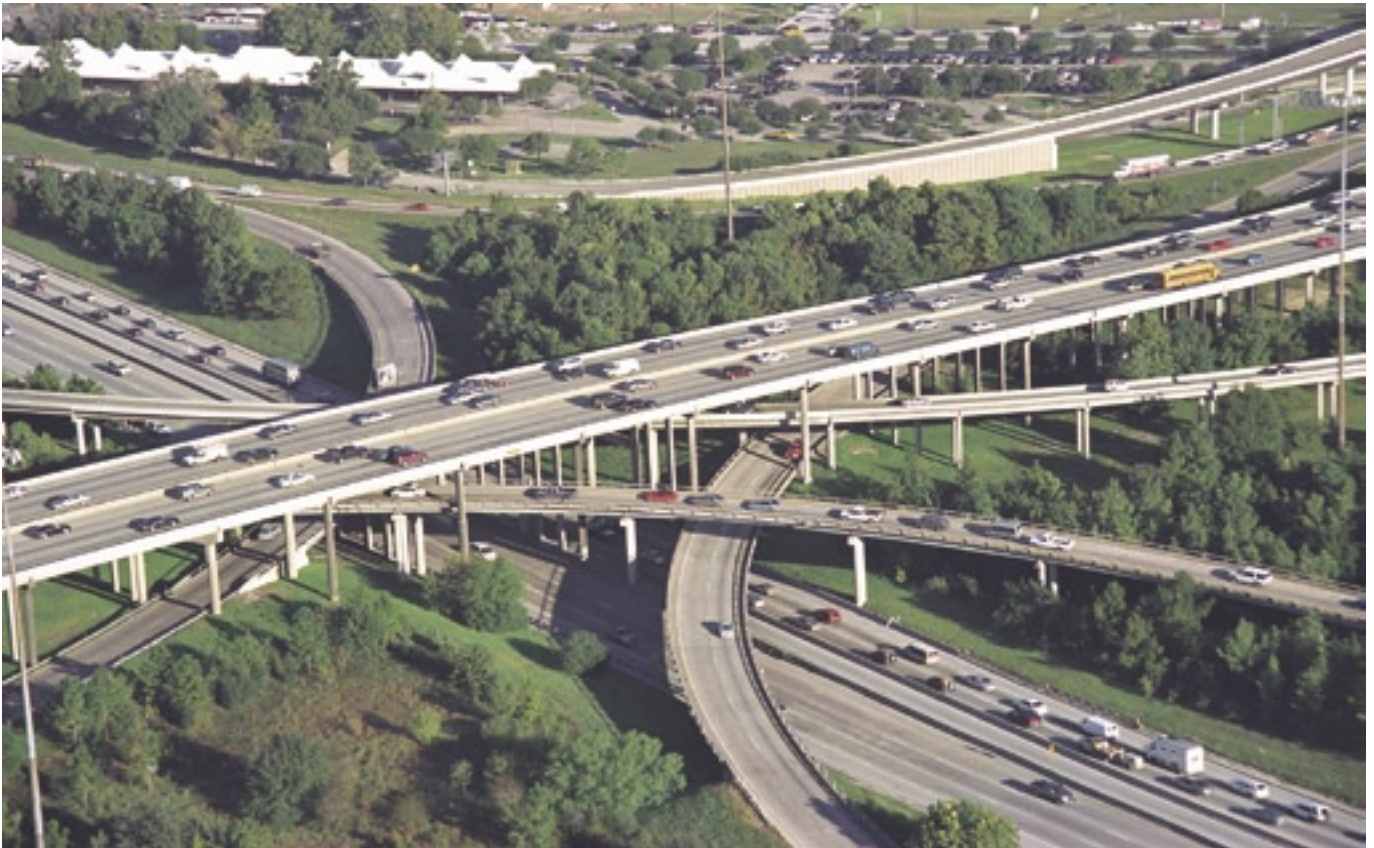
Katy Freeway-West Loop interchange, 1968-2004: In a project that began in summer 2003, this four-level interchange completed in 1968 will be demolished and replaced with a new interchange having geometrics and ramp capacities to accommodate the expanded Katy and West Loop Freeways. This will be the second replacement of a four-level interchange in Texas, following the replacement of the downtown Mixmaster in Fort Worth, a project completed in 2001. (Photo: November 2002)
