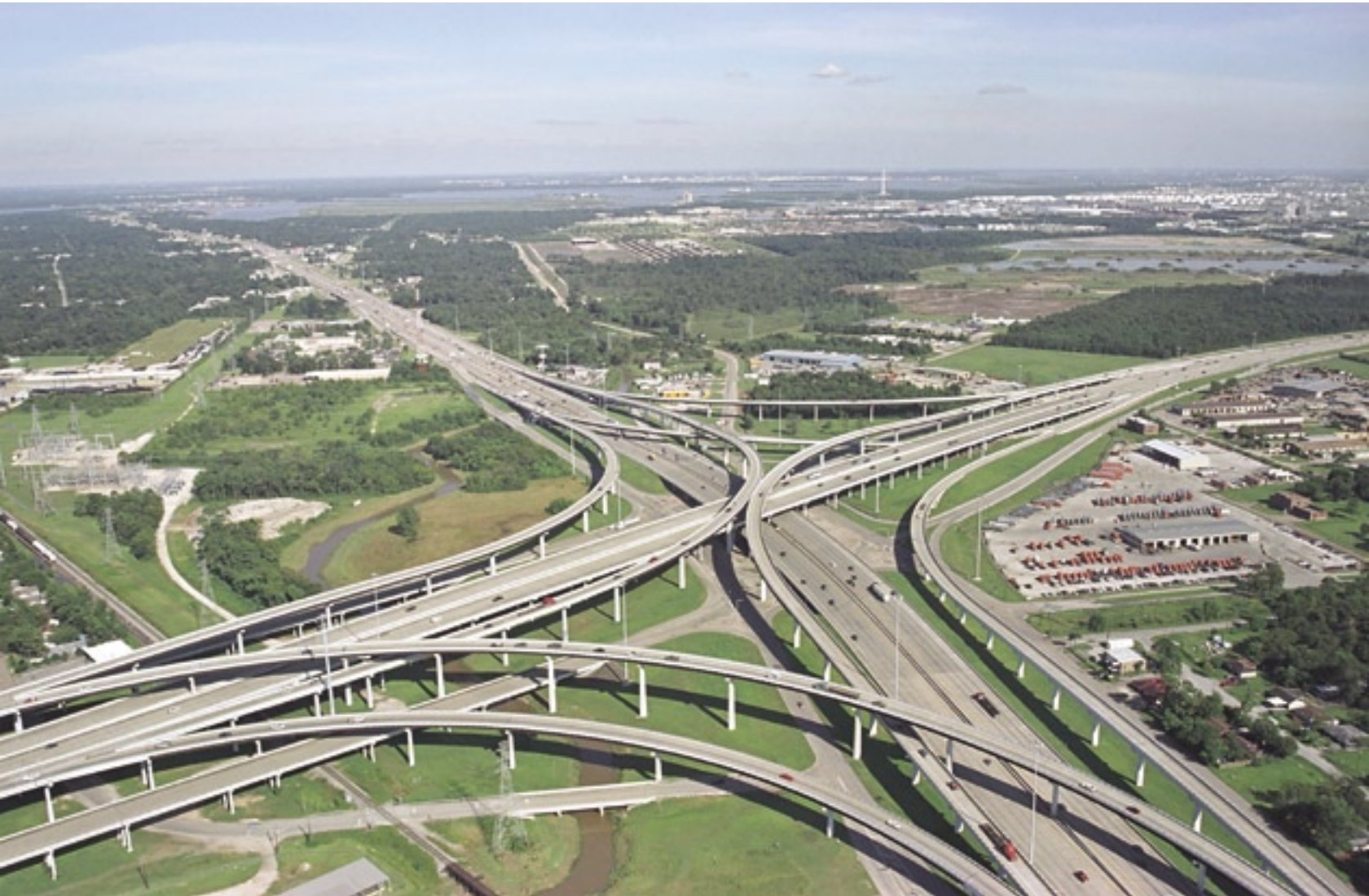
Beltway 8 interchange: This view looks southeast with the East Freeway crossing from lower right to upper left. This interchange was completed in 1994. (Photo: September 2002)
