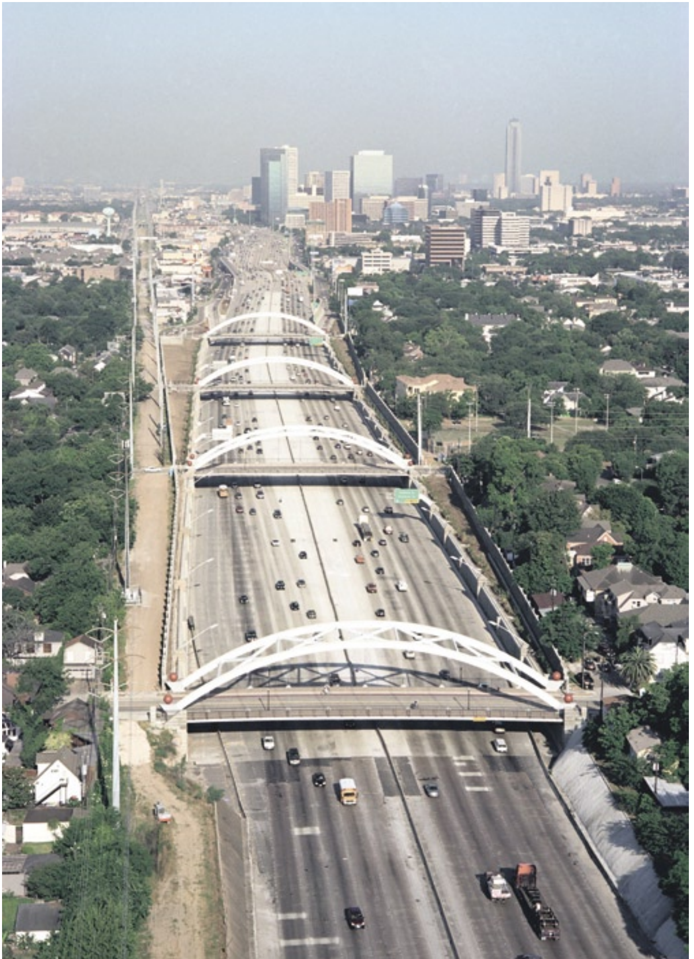
Overarching style: This view looks west along the freeway with the Mandell overpass at the bottom. (Photo: May 2003)
