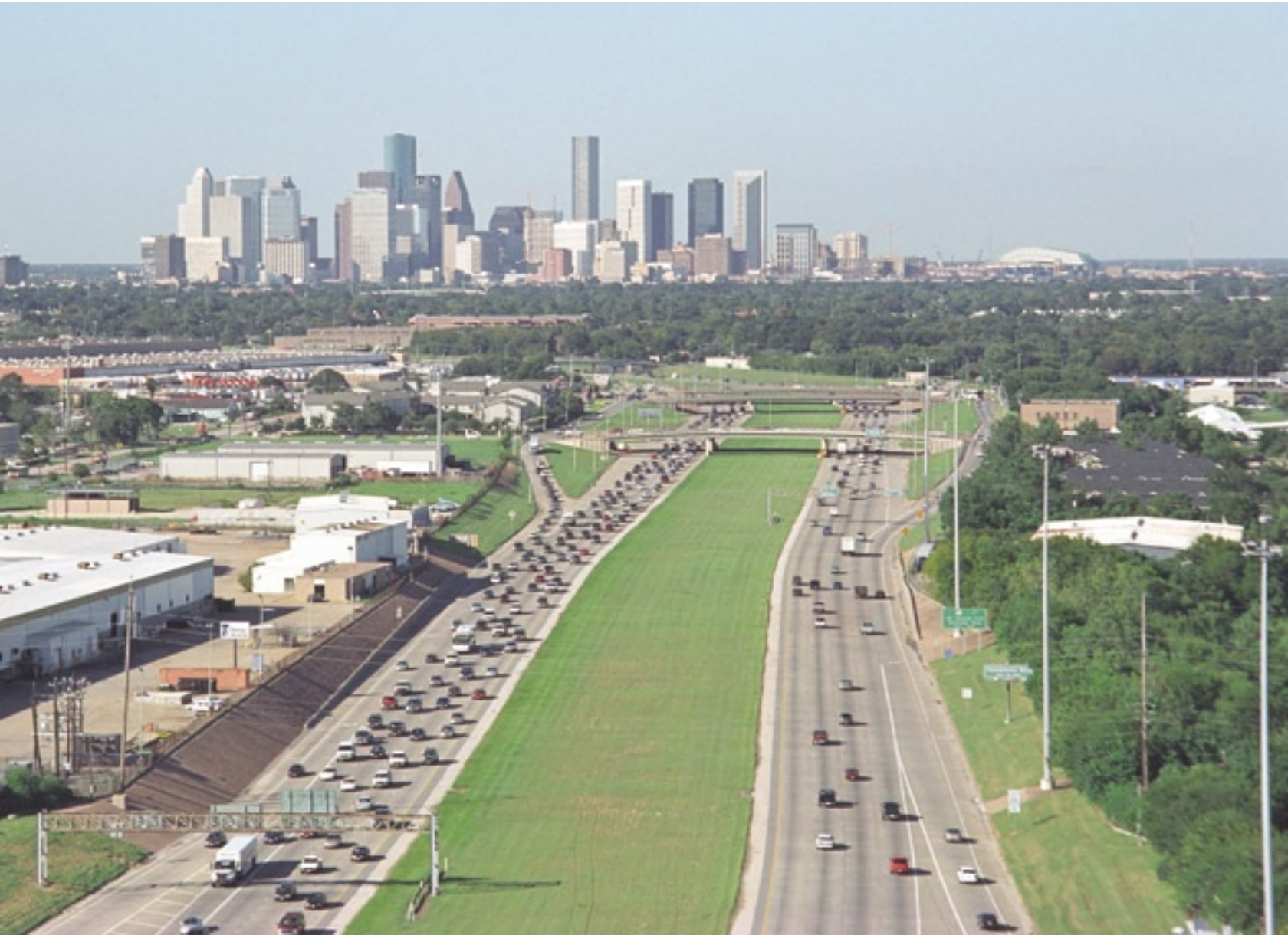
No frontage roads: The South Freeway is the only freeway in Houston constructed without frontage roads for most of its length. (Photo: September 2002)
