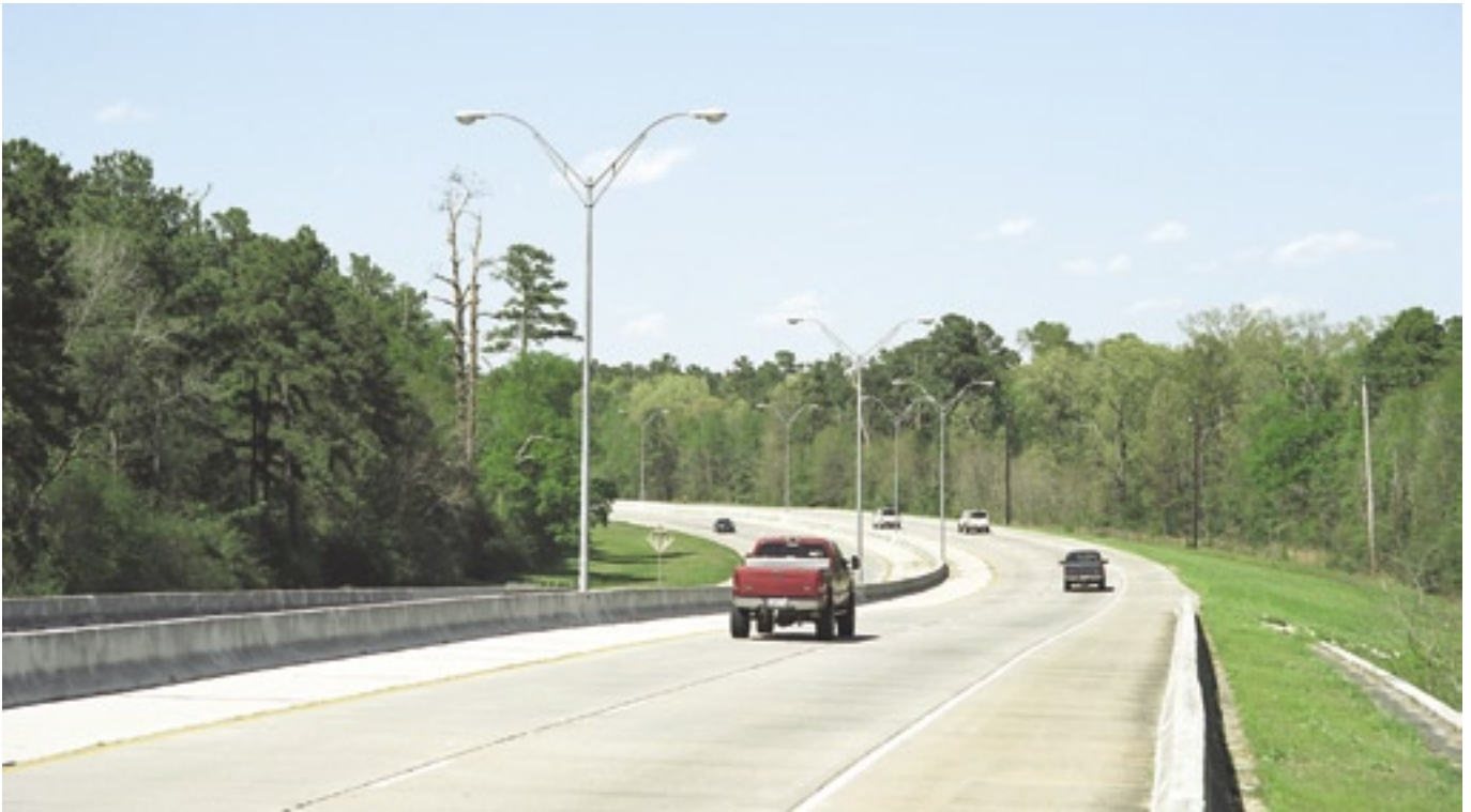
Unusual for Houston: The northern section of the Hardy Toll Road does not have frontage roads, preventing the proliferation of commercial development. Parts of the tollway are like a parkway as it passes through forests. (Photo: March 2003)
