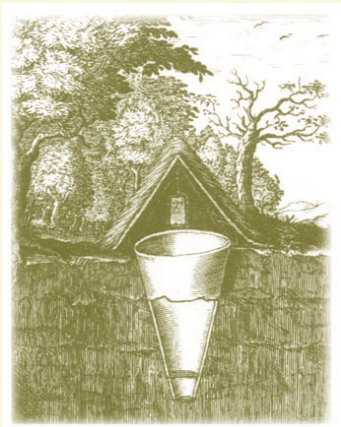
An engraving published in 1683 illustrating an Italian icehouse as described by John Evelyn. Note the conical well (presumably made of brick) with a sump and the roof of insulating thatch. (From Robert Boyle's 'New Experiments and Observations... Touching Cold.') (British Library)
