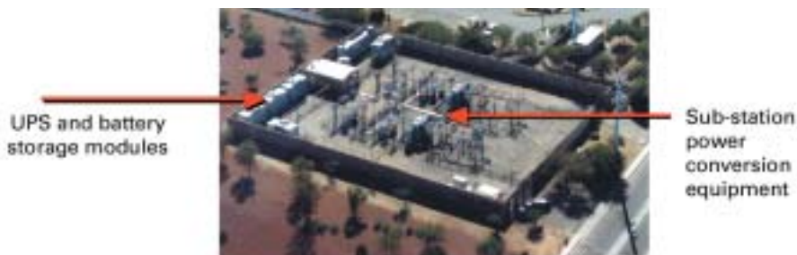
Exhibit 7.6 ES facility at STMicroelectronics, Phoenix, AZ (source: ESA/S&C PureWave)
