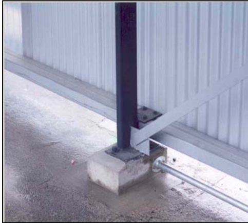
Figure 9 Origin Pacific Terminal exterior detail of base
