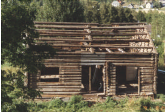
Dismantling a log home, left, and assembling a similar structure. (Photos by K.I. Edvardsen)
