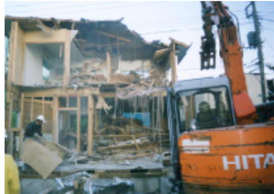
Photo 2 Wood frames demolished by machine.
