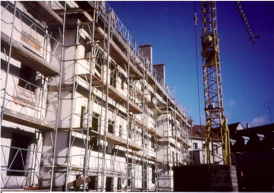
Figure 17 Dismantling in Mulhouse
