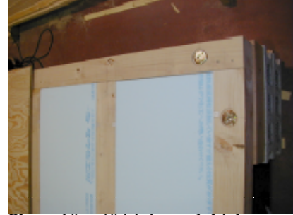
Photo 10 404 joist and thick plywood floor sheathing.
