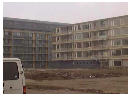
Fig 1: The old and renovated apartment building
