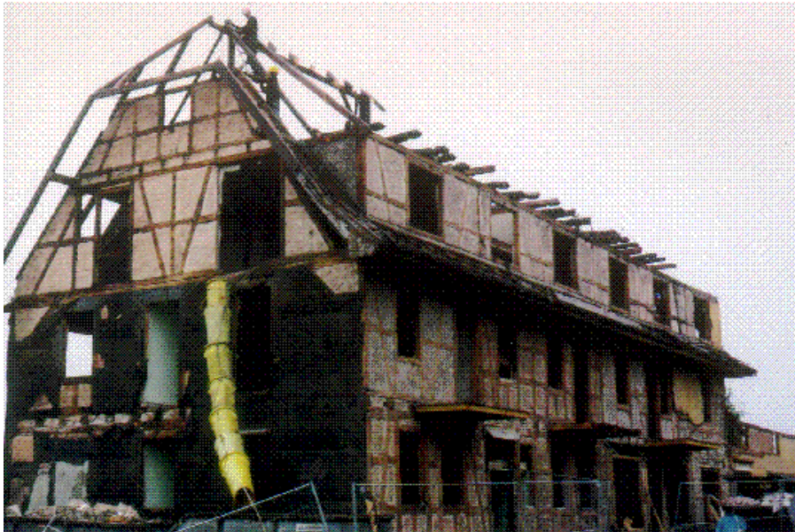
Figure 15 Dismantling of the Hotel Post in Dobel [49]
