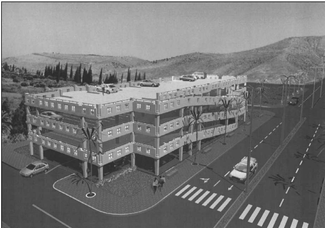
Figure 1: Computerized image of a full size parking structure designed for deconstruction (design: Villa Nir, structure: Moshe Peer, construction: Solel Boneh).
