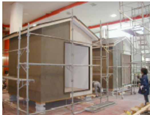
Photo 4 The test houses. Left “Improved” and right “Benchmark”.
