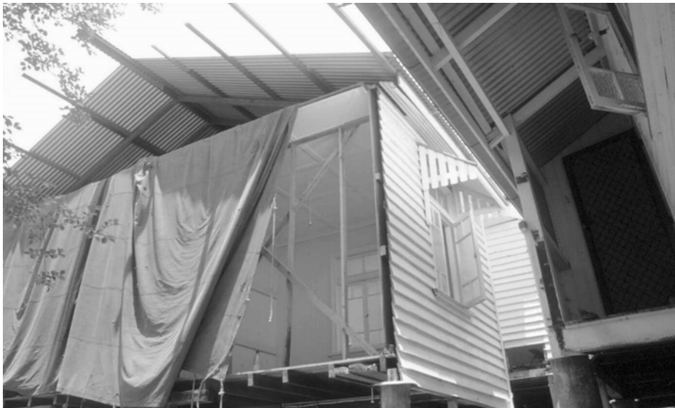
Figure 4 House during relocation – house has been relocated in two halves that are set apart to create new relationship (by Jeremy Salmon Architect).
