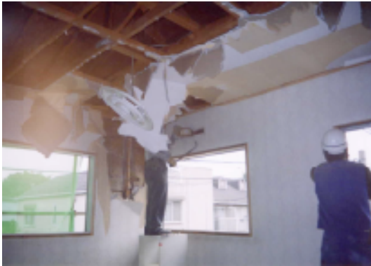
Photo 1 Gypsum boards remove by hand.
