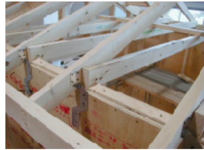
Photo 7 Joints of the framing members of the roof.
