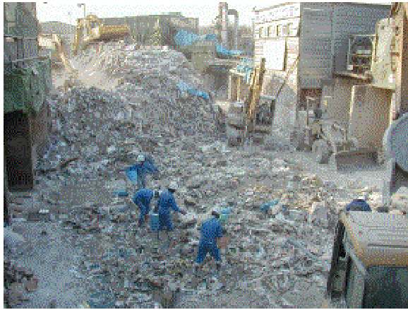
Photo10 Rough separation process of the mixed waste.
