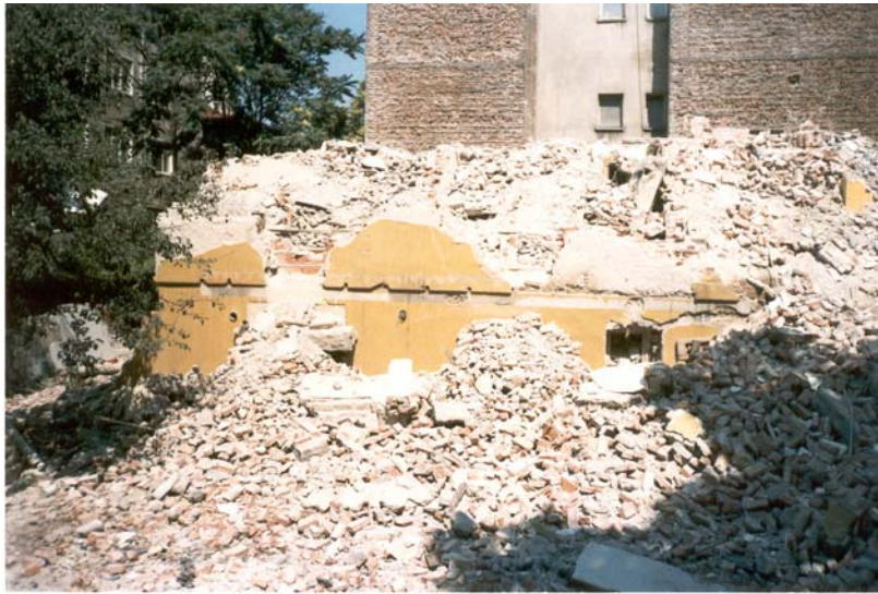
Figure 2 Rubble from the demolished building in a residential district of Ankara, has been left behind on the site.
