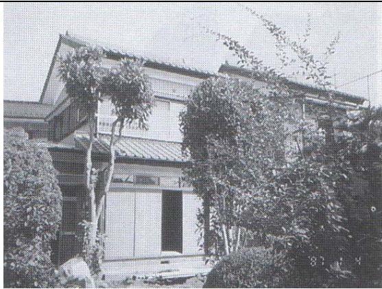
A view of the building to be demolished.
