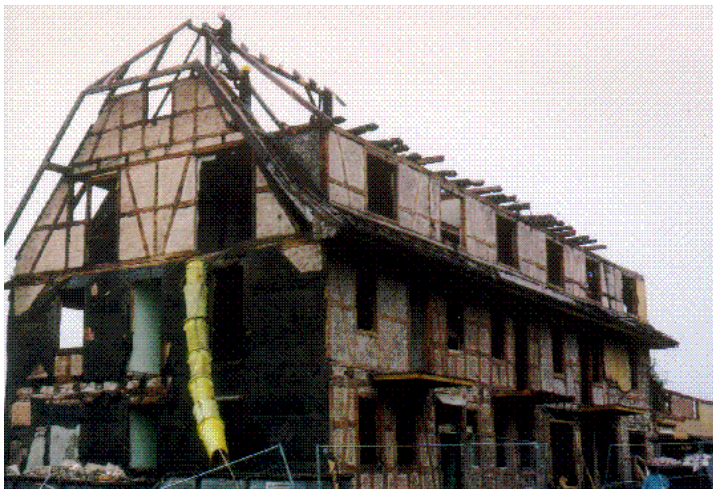
Dismantling of the Hotel Post in Döbeln
