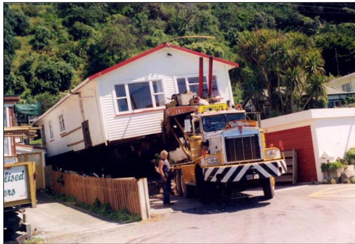
Figure 5 House leaving site on the back of a truck 69
