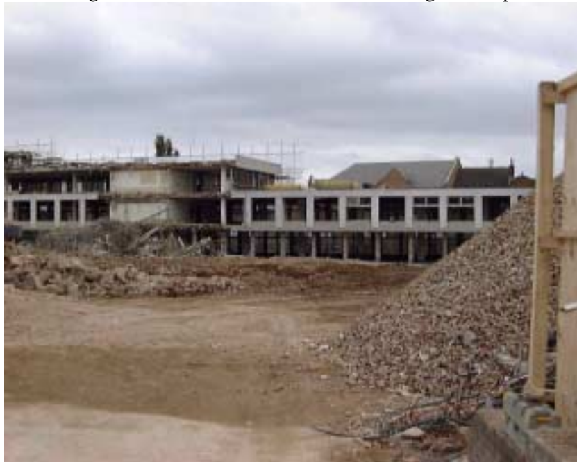
Figure 4. Demolition of structures following soft strip
