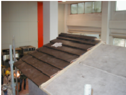
Photo 5 Roof tiles and roof felts.
