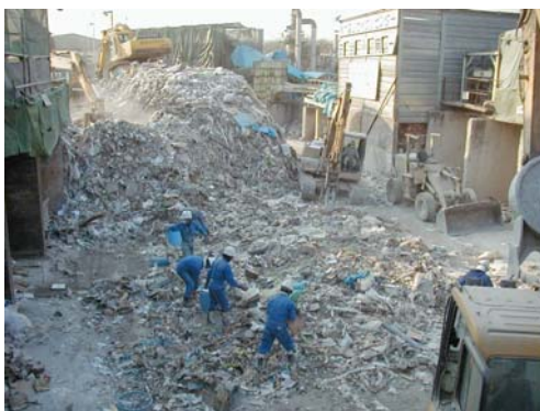
Photo 5 Segregation of mixed waste
