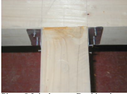
Photo 8 Joist hanger. Dual head nails are used to connect the joist hanger.
