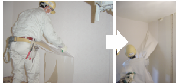
Photo 13 Wallpaper removed. Left: vinyl type wallpaper. Right: cloth type wallpaper. Cloth type wallpaper can be easily removed compared with vinyl type wallpaper.
