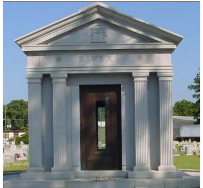
The mausoleum of Governor E.D. Rivers was constructed as a replica of the Georgia State Capitol ca. 1968.
