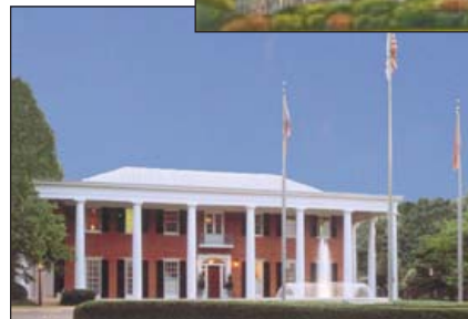
The Victorian house on Peachtree Street was home to 17 governors from 1870 - 1921. The mansion in Atlanta's Ansley Park was used from the 1920s until 1968, when the current Governor's Mansion, located on West Paces Ferry Road in Atlanta, was completed. Image of the current mansion from "The Georgia Governor's Mansion" brochure, Office of the Governor.
