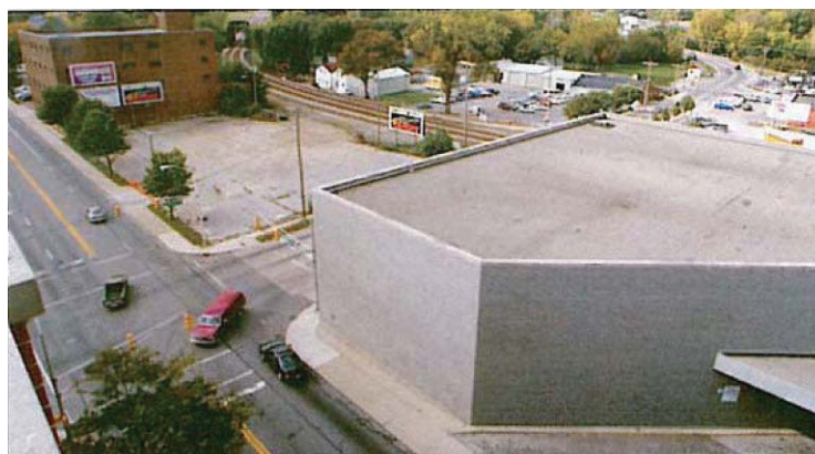
Fort Wayne Newspapers; new press hall will go up on the Main St. site of the lot and building (top left) west across Sherman Blvd. from its existing plant.
