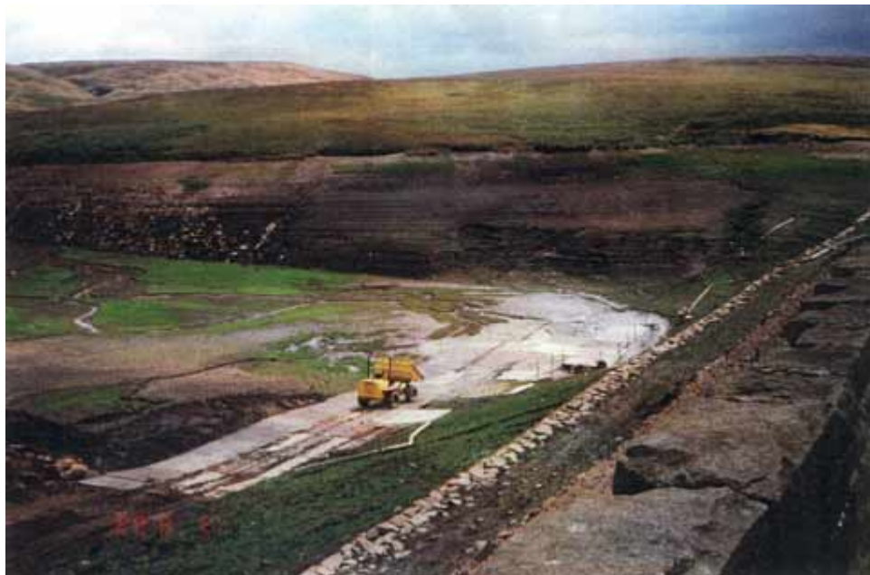
Removing Sediment from around low level outlet (reservoir in peat catchment)
