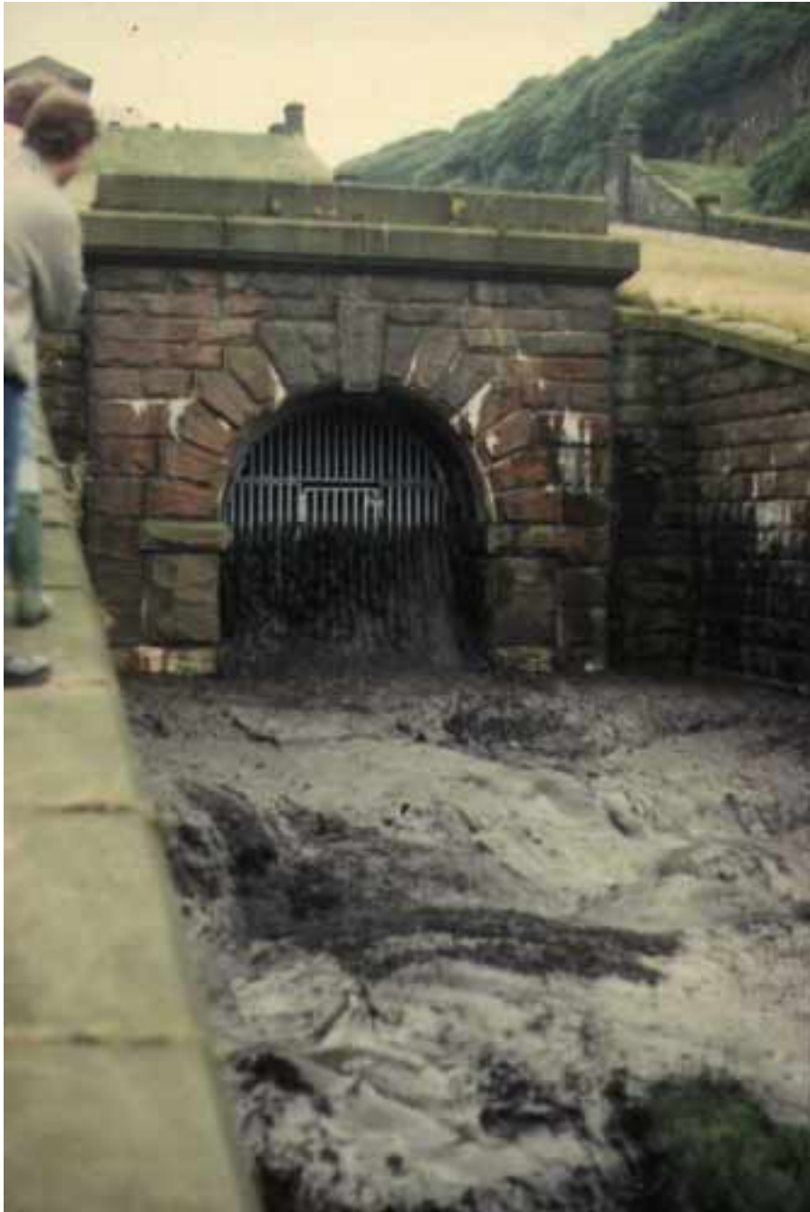
Progress of Scour valve test, Blakeley Reservoir, October 1985
