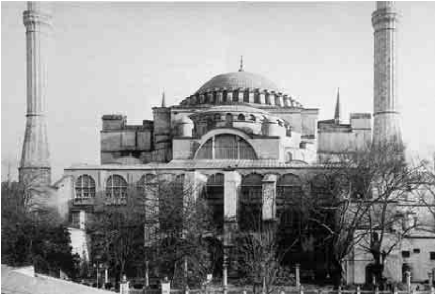
3. Istanbul, Santa Sofia, facciata nord-ovest (da R. Mark, A.S.Cacmak, Hagia Sophia from the age of Justinian to the present , Cambridge 1992).
