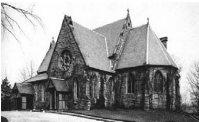
The south facade, including a view of the apse, shortly after the completion of the building; note the absence of the belfry and the enclosure of the transept porch
