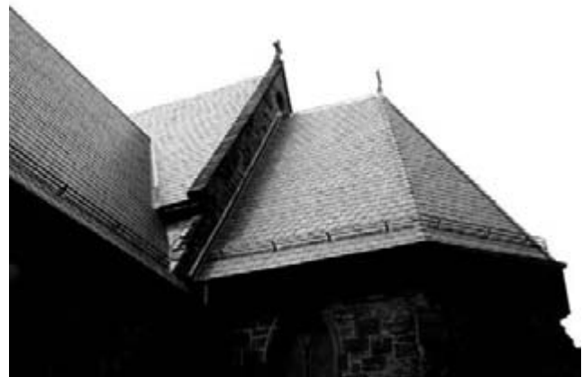
The newly restored roof of the apse
