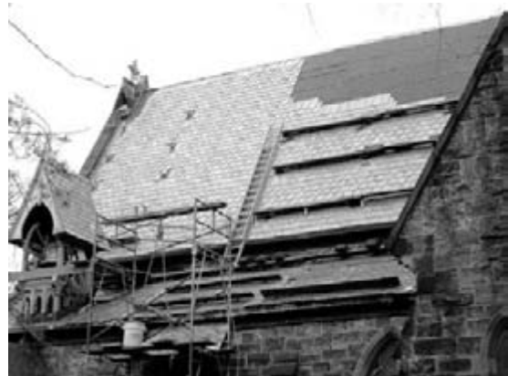
The restoration under way
