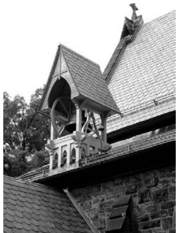
The restored belfry
