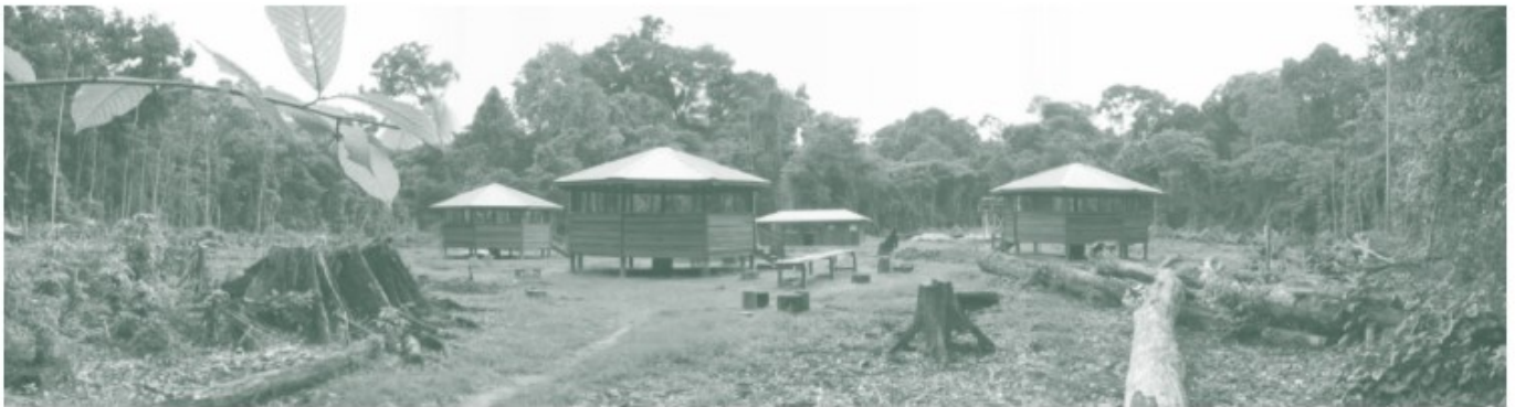
Above: Turtle Mountain Campsite under construction
