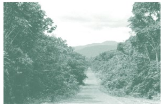
Section of the Iwokrama Road Corridor
