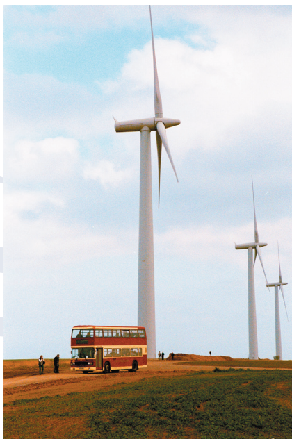
Out Newton wind farm © E. ON UK Renewables
