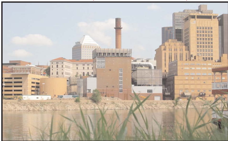
Fig.1. District Energy Saint Paul customers are now heating and cooling their buildings with "green energy" produced at a new CHP plant adjacent to the company's downtown facility. Photograph credit: Nancy Toohey.
