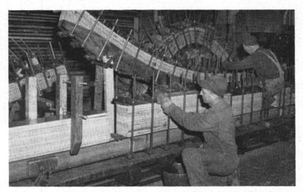
SPECIAL glues, hydraulic presses and clamps enable naval shipyards to make big timbers out of little boards and then bend them like so much cardboard.
