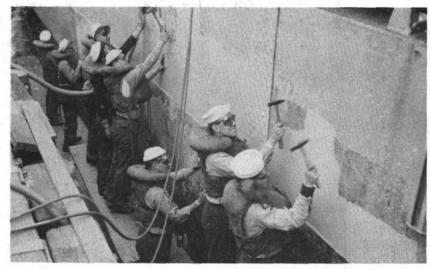
SHIP'S FORCE turns to in a paint chipping assignment. Life jackets and goggles must be worn for this work. Before long, vessel will have fresh paint.
