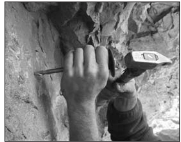
Drilling anchors on Faded Glory. Brent Edelen
