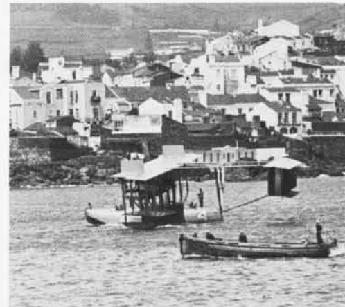
On May 20, 1919, the Navy's NC-4 landed at Ponta Delgada on the island of Sao Miguel before completing the world's first trans-atlantic crossing.
