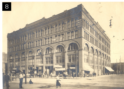
Southeast corner 4 th and Court Streets
