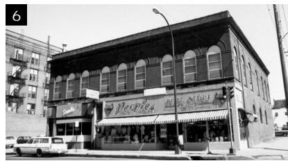
Northwest corner 4 th and Court Streets
