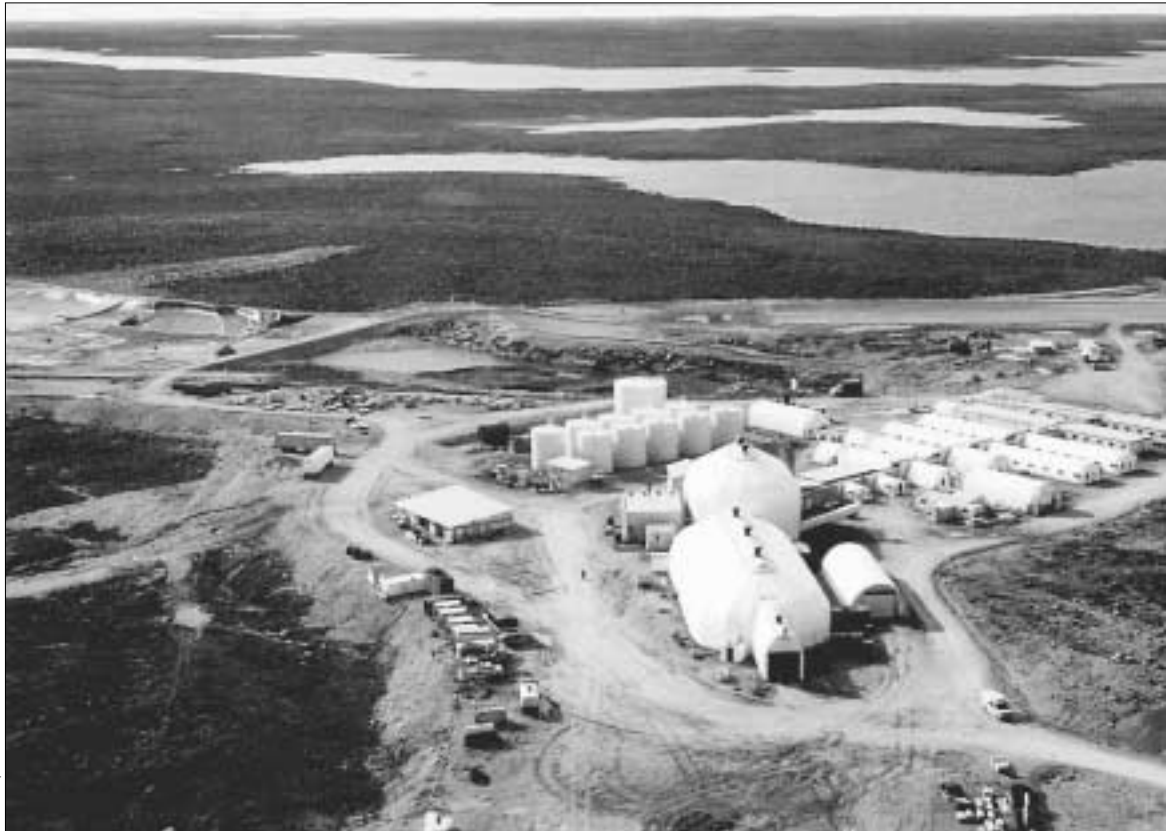
BNP/Dia Met bulk sampling plant at Lac de Gras, Canada
