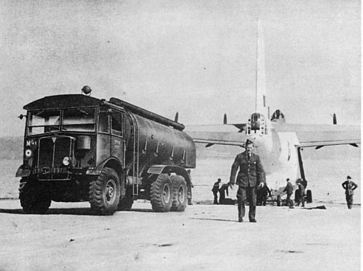
Not only a fuel tanker but a towing vehicle as well. This A.E.C. R.A.F. tanker accomplishes with ease the secondary task of towing "Sunderlands" ashore at a Scottish coast station.
