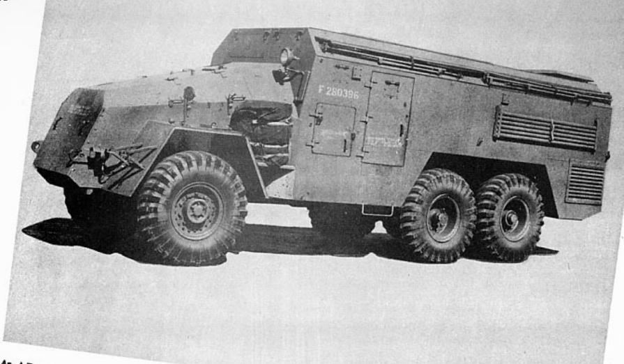
An A.E.C. 6-wheel drive armoured command vehicle of which 151 were built for service overseas.
