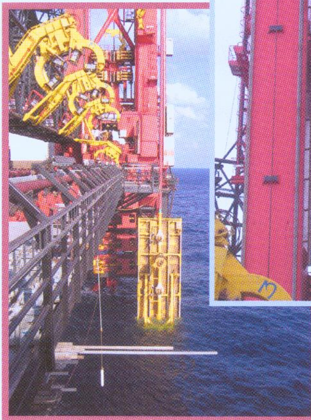
Figure 1. Heavy inline structure ready to be submerged.
