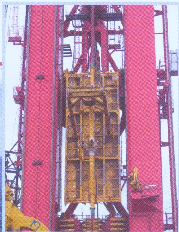
Figure 2. Heavy inline structure installed in J-lay tower.
