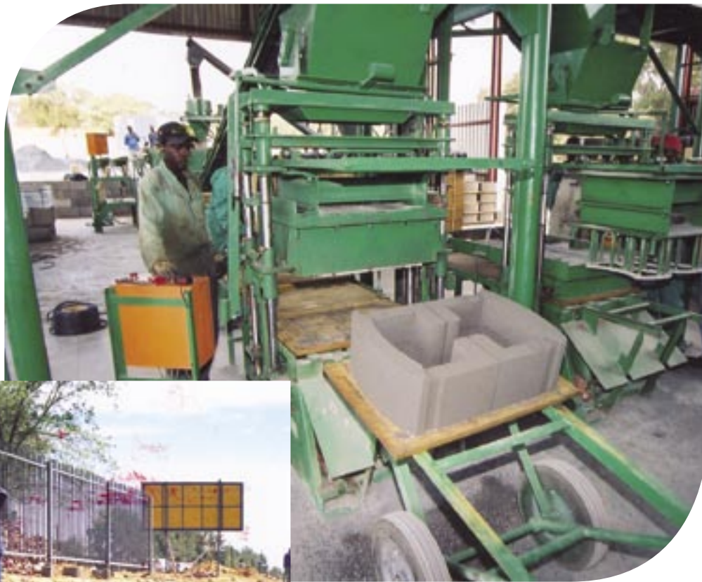
(Above) Concrete retaining blocks come off the production line at the recently commissioned concrete retaining block factory in Chloorkop, Gauteng
