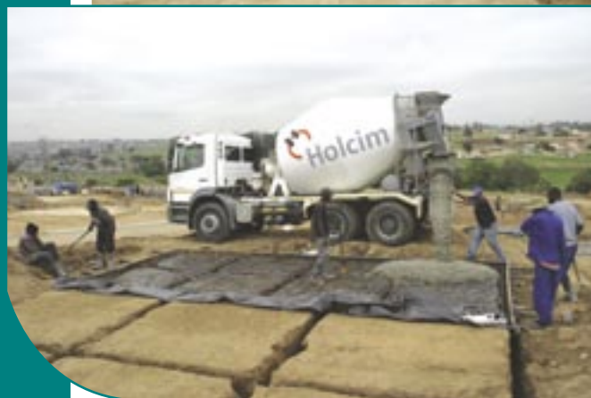
The soil pads under the entire foundation are 'wrapped' in plastic sheeting to ensure that no rising damp can get through the slab and the steel reinforcing is hand-fixed to suit the shape and beam layout of each house.
