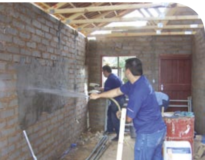
The interior walls are prepped before product application.
