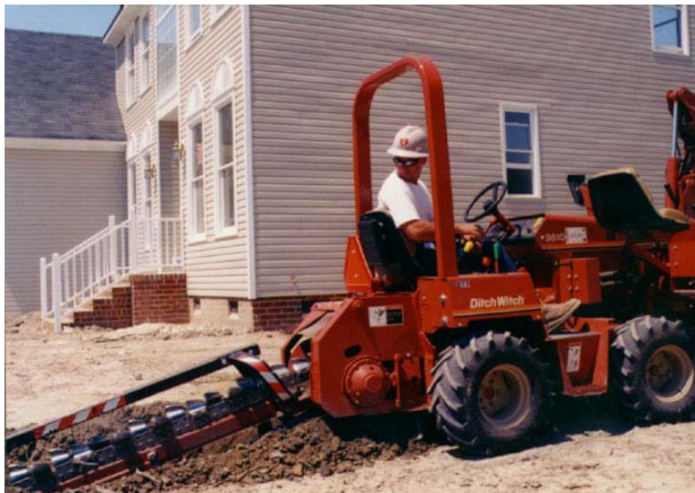
Figure 11: Typical Trenching Operation for Residential Services
