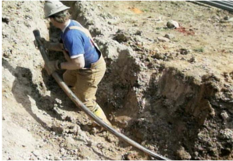
Figure 12: Installing Flexible Conduit in an Open Trench
