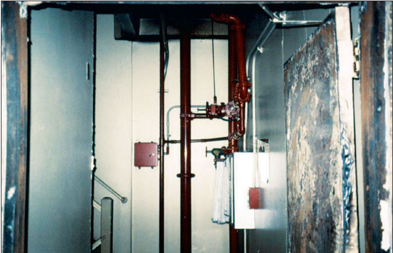
Figure 4-16 Looking through the door into the undamaged stair tower in WTC 5.
