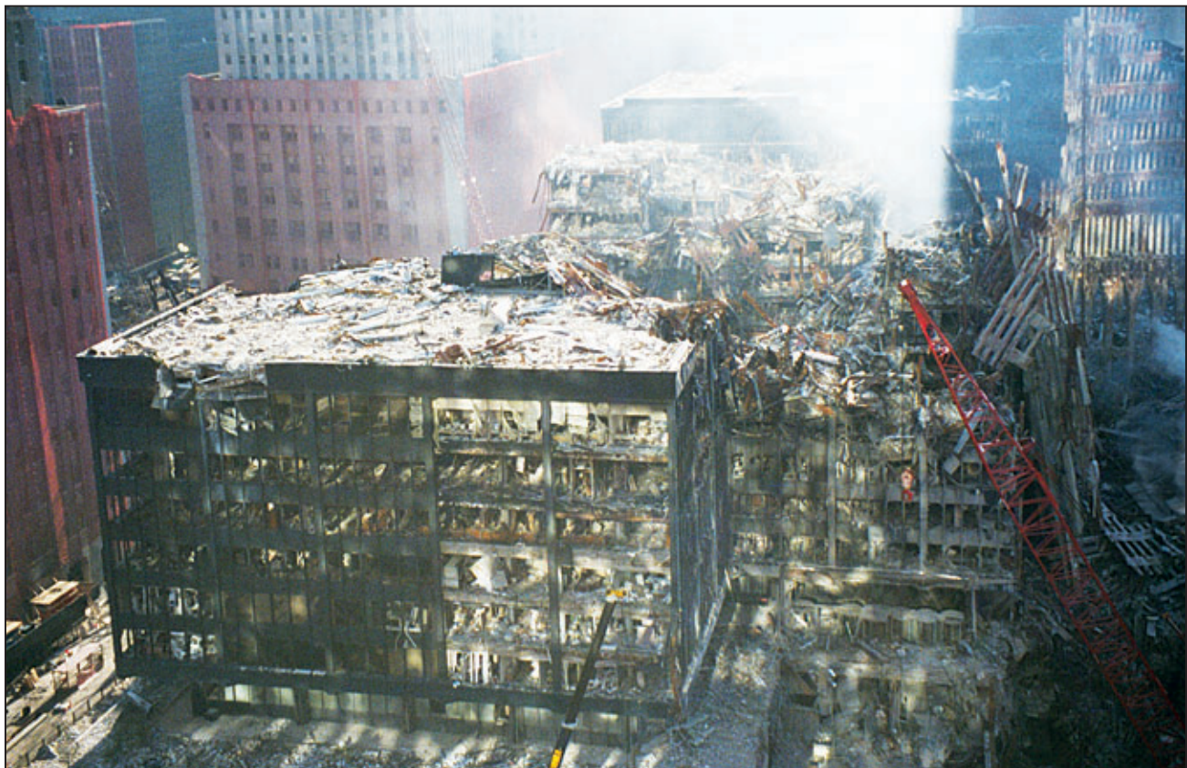
Figure 4-9 Impact damage to WTC 6.
