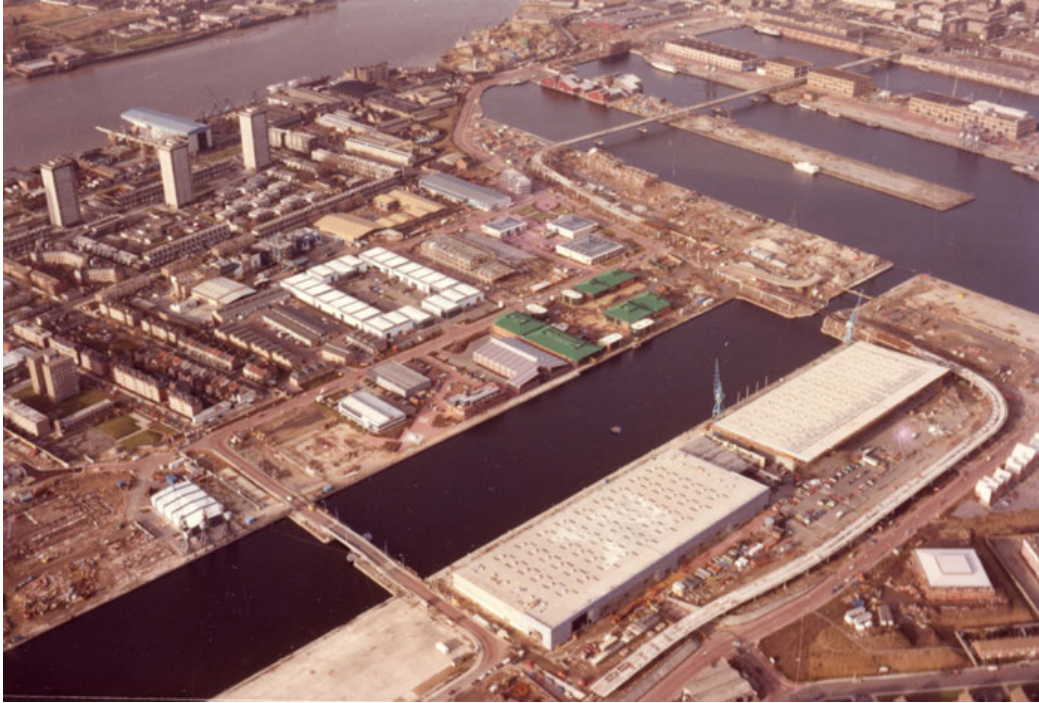
Photo 6 - DLR track under construction over West India Docks Millwall Cut, mid-1980s
